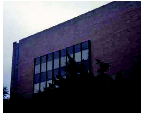
Side Vertical Façade of NAAB
