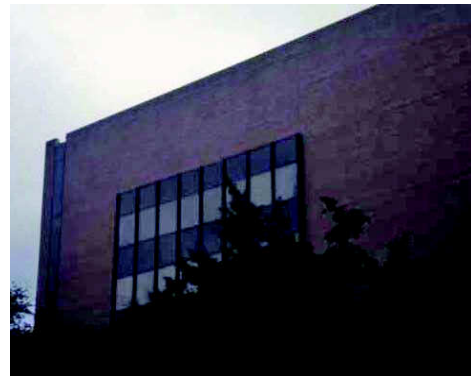
Side Vertical Façade of NAAB
