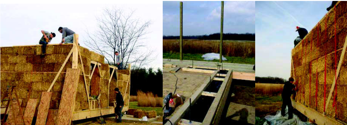
Figures 10-12: Installing the top plates on the bale walls; platform prepped to receive the bales; pre-compressing the bales;
