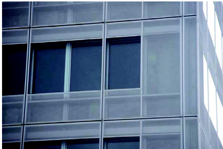
Figure 5: A well integrated double facade that supplements the performance of a building with: a shallow floor plate, concrete mass, radiant cooling, ground water wells, displacement ventilation, and an earth tube. Münchner Tor, Munich, Germany, 2003. Allmann, Sattler, Wappner.
