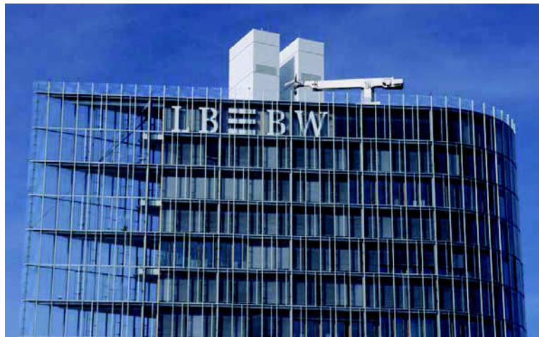
Figure 6: The double facade as icon. With a teardrop shape in plan, much of the outer glass leaf has no occupied space behind it. Landesbank Baden Wurtemberg, Haus 5+6, Stuttgart, Germany, 2004. Wohn Mieslinger Architekten.
