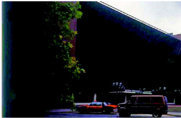
Front Façade of NAAB with 30° Tilted Façade
