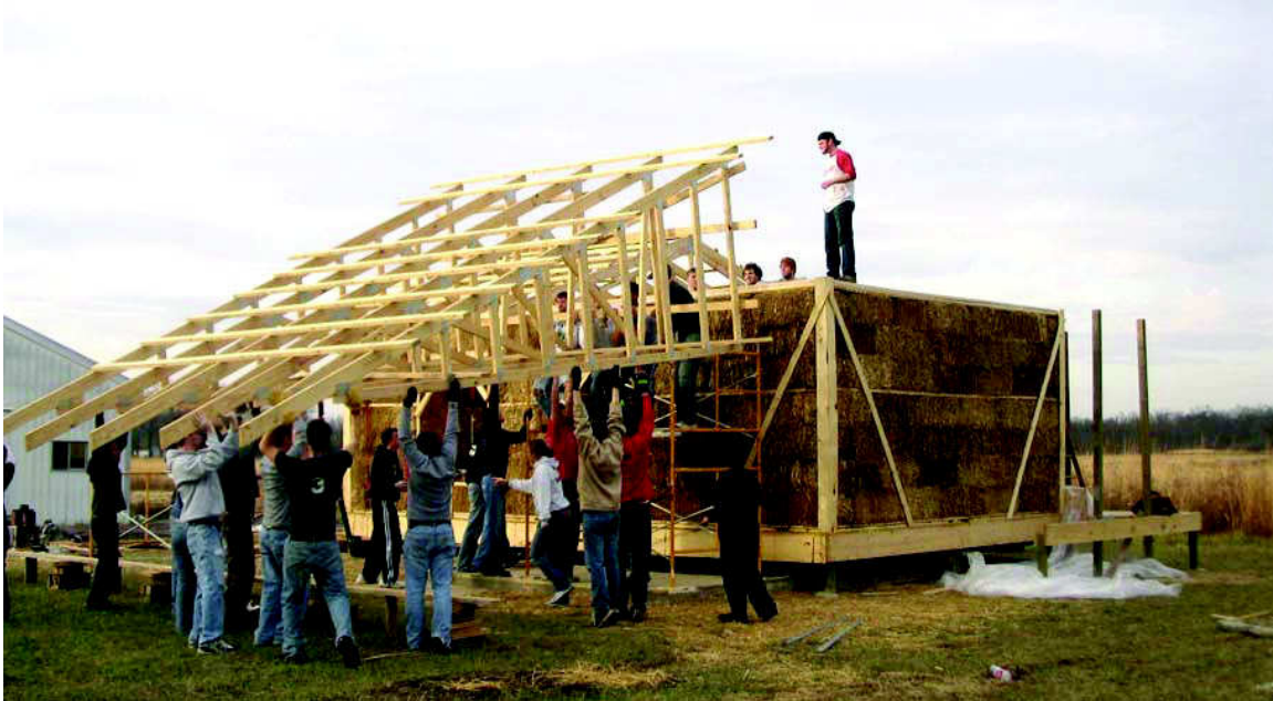
Figure 13: the community "truss raising"
