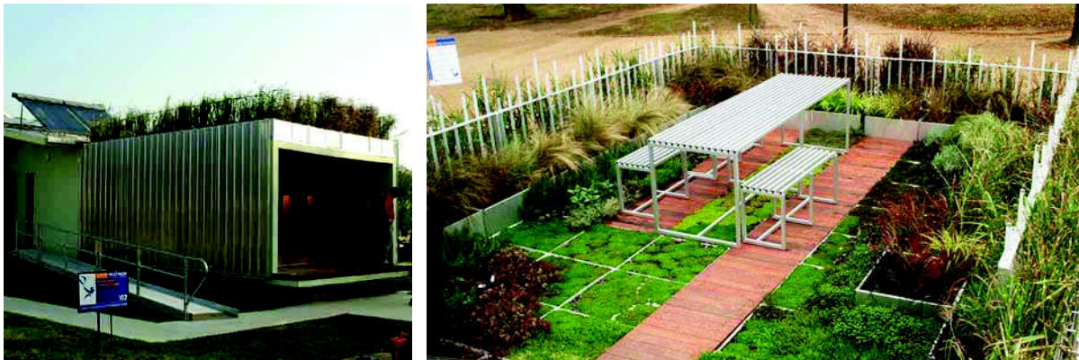
Figure 1: 2005 Rhode Island School of Design Solar Decathlon House with a green roof for outdoor dining.
