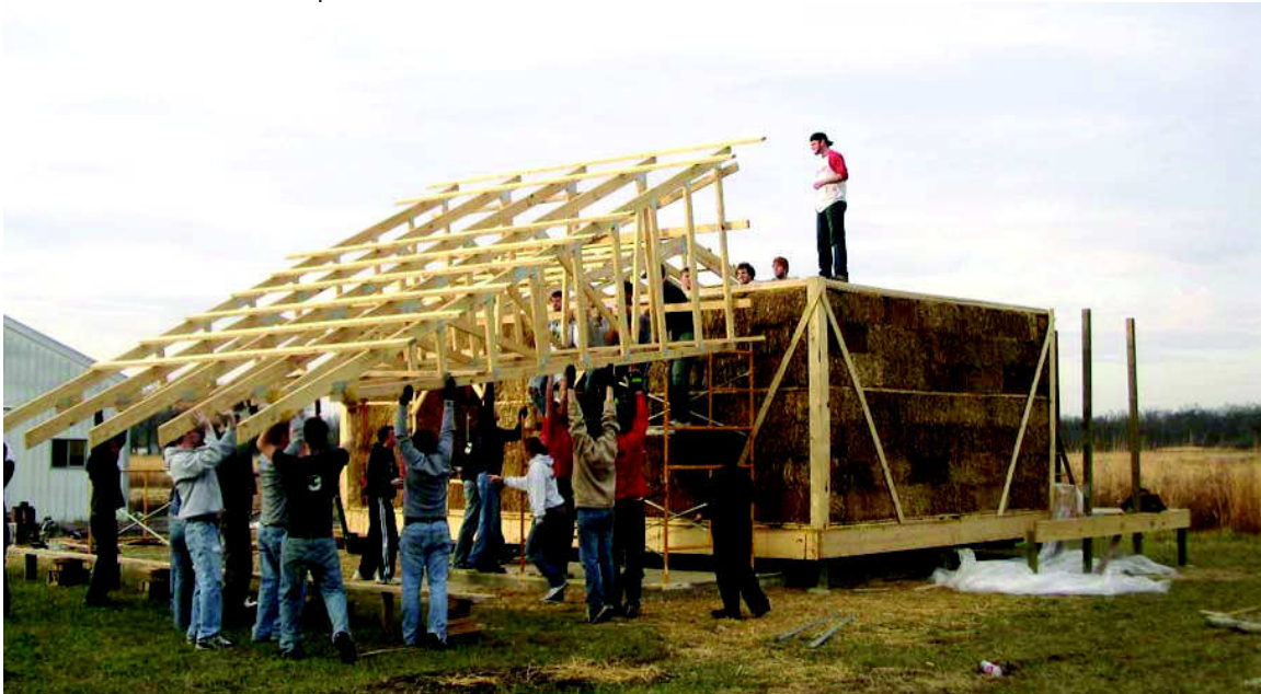
Figure 13: the community "truss raising"
