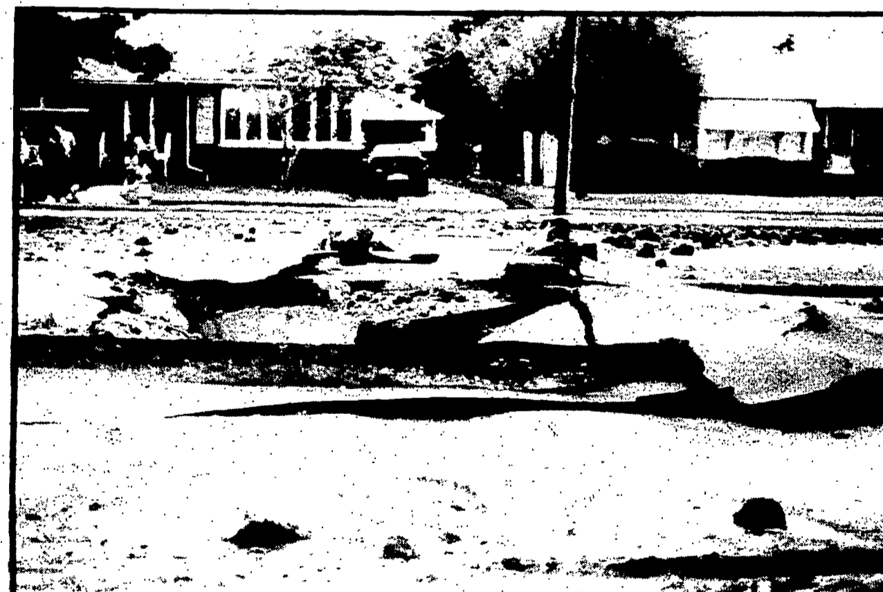
An explosion last Friday evening buckled the pavement and formed a crater on Oakton Street near the intersection of Waukegan Road. The blast was the result of the hydrostatic testing of a 36" gas pipe line for underground leaks. No injuries were reported in the incident but Oakton was closed to traffic during the cleanup.
