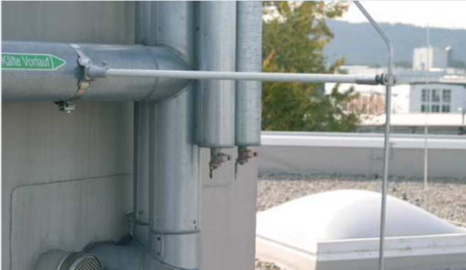
Spacer with attachment, fixing bush and tensioning strap
