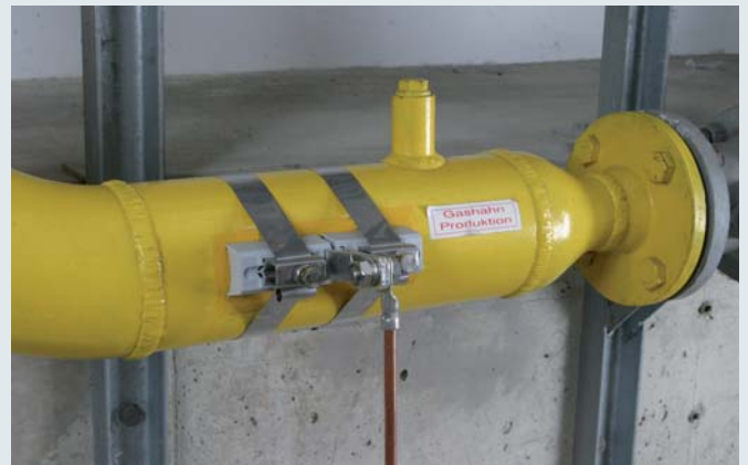
Pipe clamp for electrical contacting of pipes in hazardous areas for implementing of lightning equipotential bonding according to IEC/EN 62305-3 (EN 62305-3)
