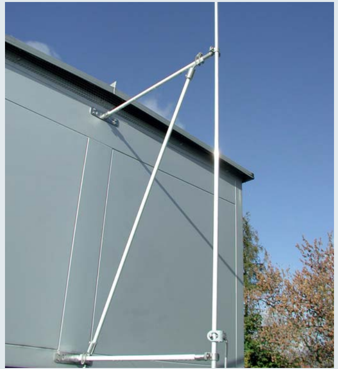
Variable range of supports for conductors and air-termination rods for keeping the separation distance according to IEC/EN 62305-3
