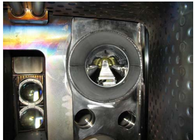
Figure 4: View of the Storage Cask through the dedicated port from inside the Tokamak
