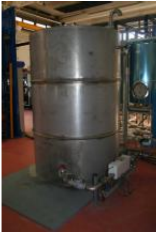
Figure 3: Water buffer tank
