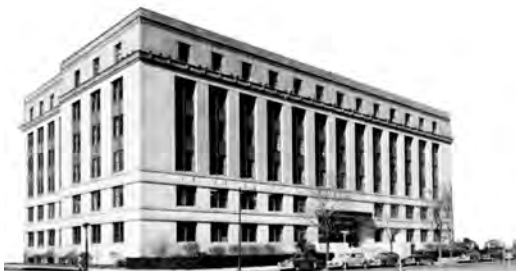
Figure 2. Envelope condition prior to retrofitting
