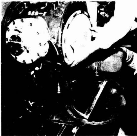
Figure 1a — Regenerator Core Removal
