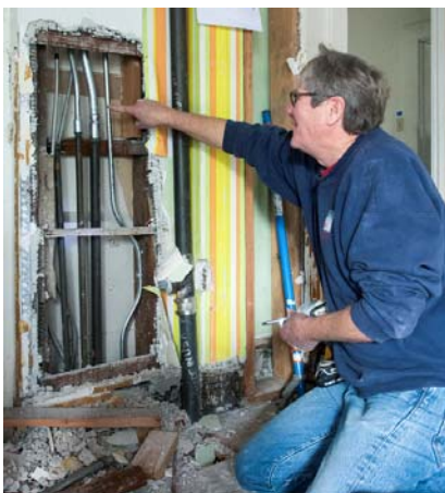
Kevin upgrades the electrical service.
