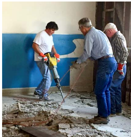
Cliff, Walter, and Larry performing final demolition in shop area.
