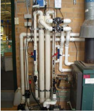
Two ozone pumps and hydro-kinetic custom-designed and built mixing vessels. Ozone is injected from the two OzoneSwim generators via the 2 vertical venturis – one gram/hour each
