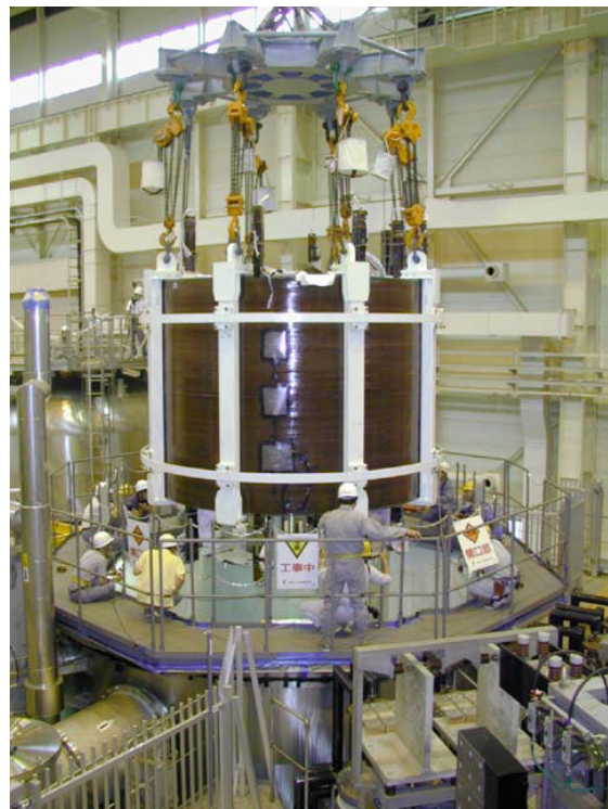
Figure 1.5.2-1 CS Model Coil The outer module being placed outside the inner module which has already been installed in the vacuum chamber.
