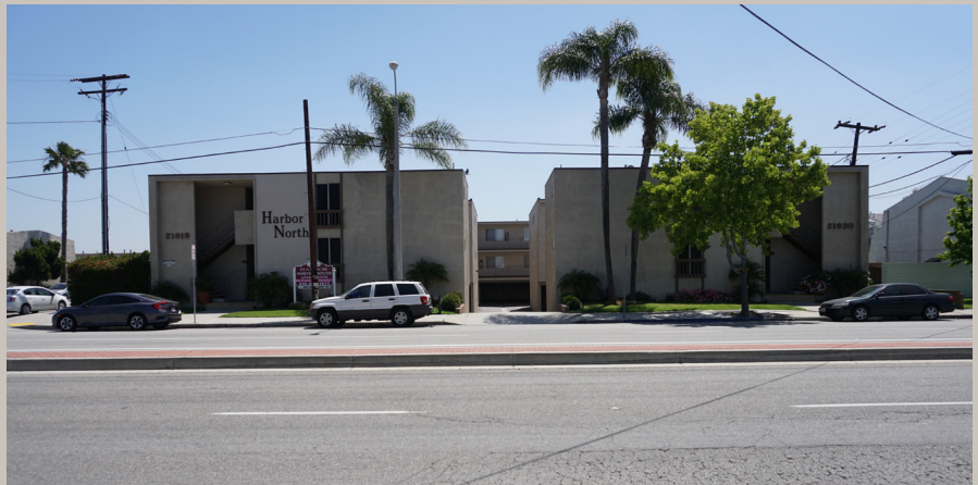
6_Multi family residential building across the street
