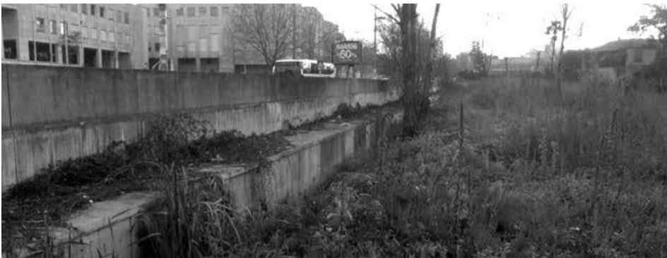
Figure 4. The existing watercourse flows in a box culvert.
