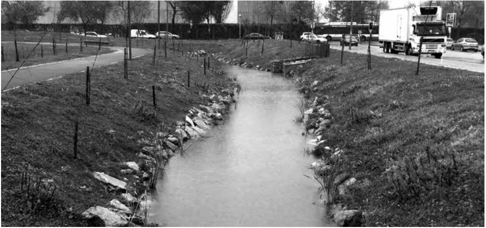
Figure 5. The watercourse currently flows in the open air. The section is able to store water during a storm event.
