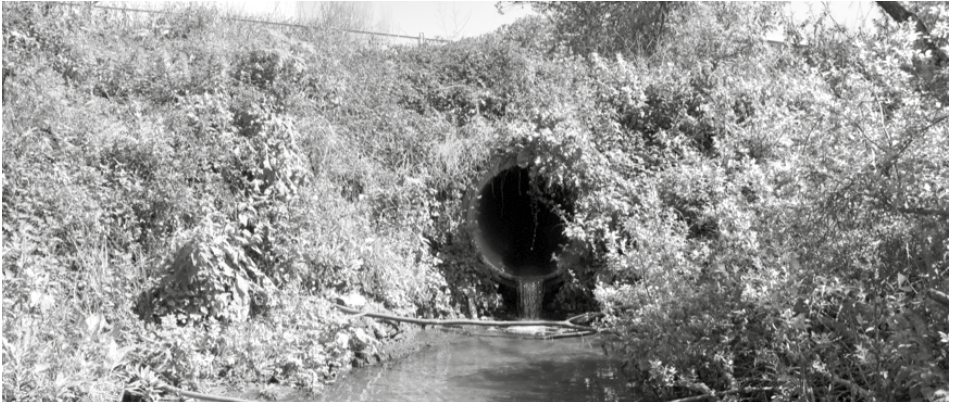
Figure 8. Asprela stream coming out of an underground concrete channel.
