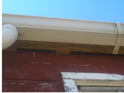
Figure 6: Typical wrap-around strap attachment to fascia board.
