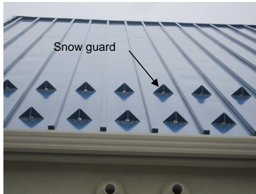
Figure 11: Typical snow guards to prevent snow and ice slides
