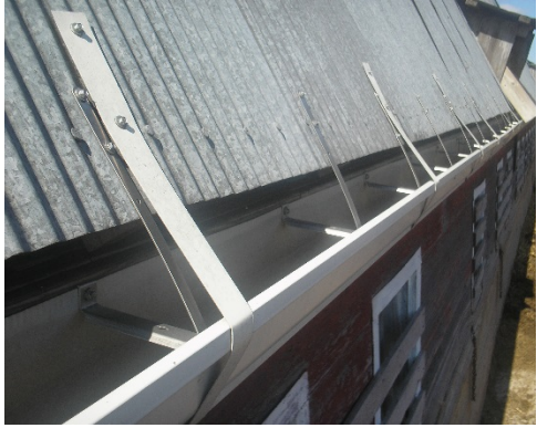
Figure 5: Typical wrap-around strap attachment to roof.
