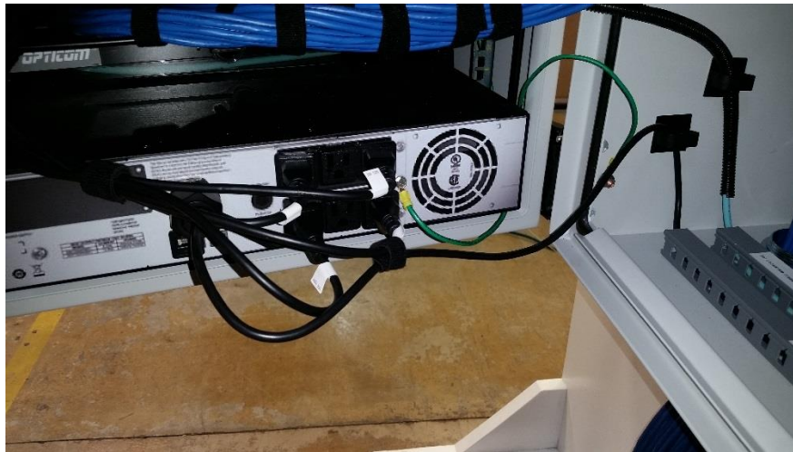
Figure 23: UPS cable routing
