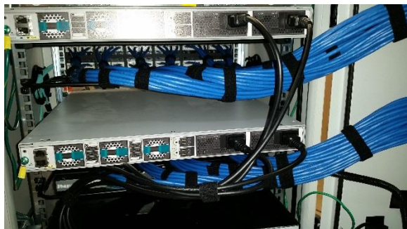
Figure 26: Switch Power Cord routing and Tak-Ty.
