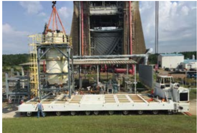
Figure 2: Relocating 10,000-gallon tank to TS 116.
