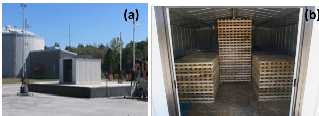
Fig. 136. Photograph of (a) steel Large shed setup and (b) the steel Large shed with high fuel loading of six 6-A cribs.
