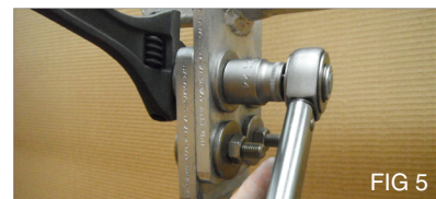
Fig B S/S OR HDG BOLTS AND NUTS WITH LARGE SERIES LOAD SPREADING WASHERS AND DOUBLE NUTS
