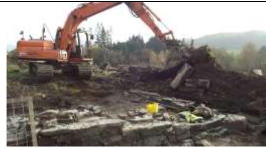
Plate 3 removing tree stumps
