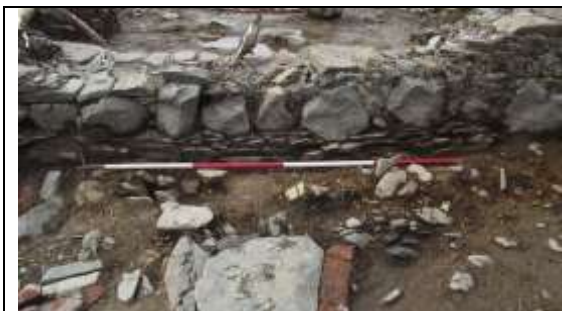
Plate 27 a. Showing basal course of gable wall of Area 3. Looking SW.
