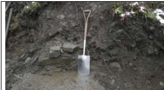
Plate 52. Showing wall at base of Trench No 1.
