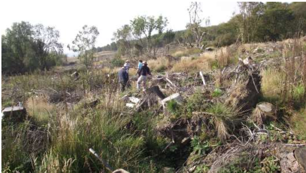
Plate 1 showing site before work began, looking SW. Compare with Pl 49a
