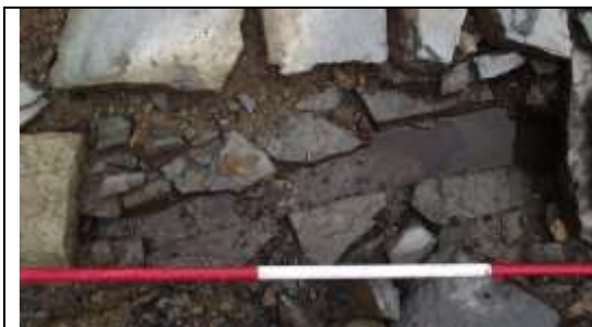
Plate 12. Showing drain in Area 1 with cover stones removed
