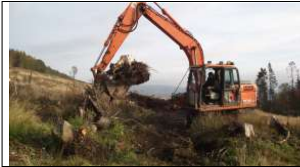
Plate 2 removing tree stumps
