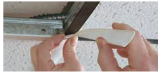
APPLYING GRIDMAX OVER T-BAR SUSPENSION GRID SYSTEM
