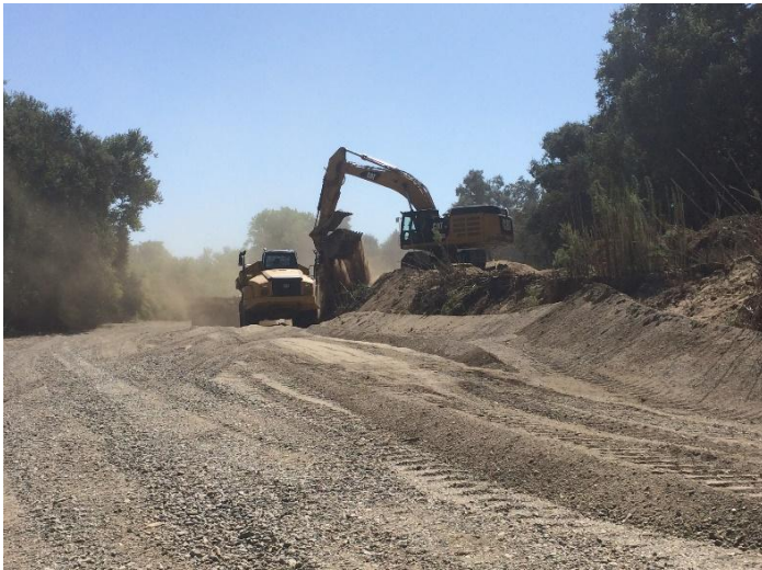
Figure 2-3: DWR Channel Improvements
