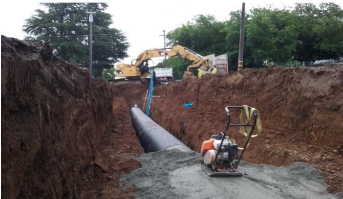
Figure 2-1: Los Molinos Drainage improvements
