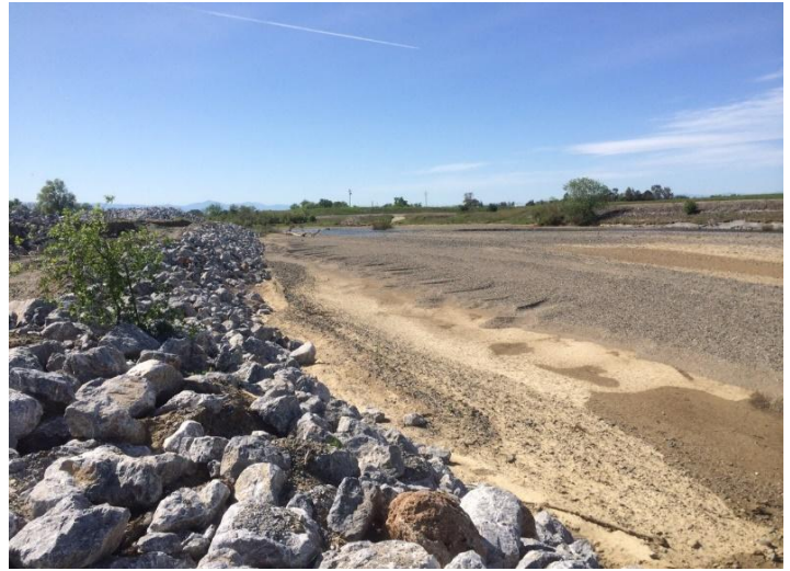
Figure 2-2: Elder Creek Improvements looking upstream after temporary repair
