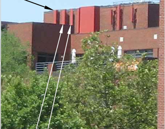
DETAIL OF EQUIPMENT
