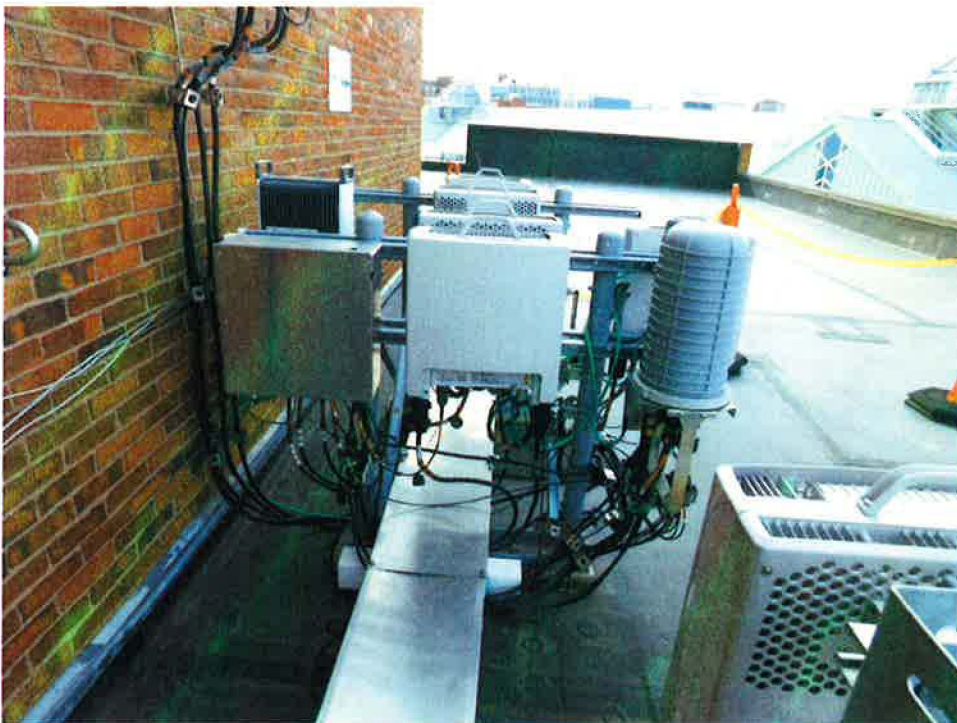
Photo 4: Sample photo illustrating the existing non-penetrating ballast mounts.
