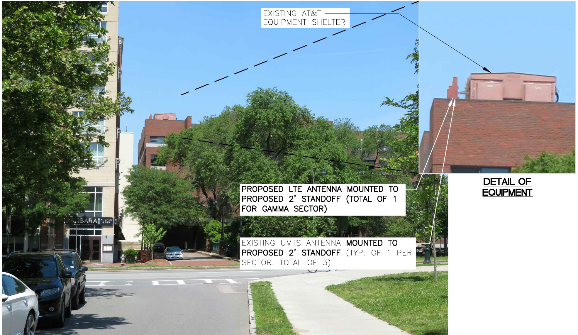
VIEW NORTHWEST FACING BUILDING FROM EDWIN H LAND BLVD
