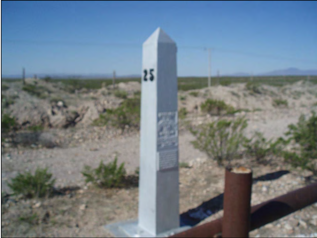
Figure C5. Overview of International Border Monument 25 facing south-southwest.
