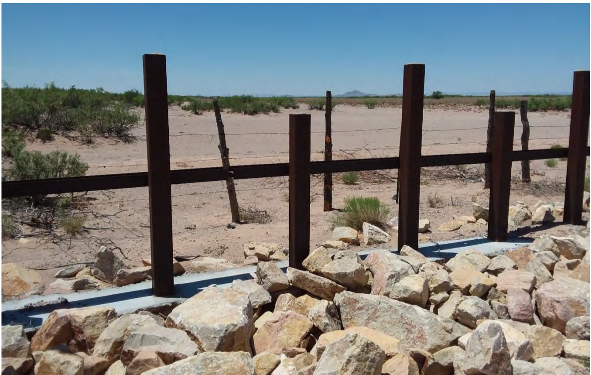
Figure 35 Photo Point K2, looking downstream into Mexico.
