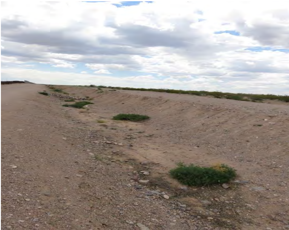
Figure 2. Artificial drainage trench
