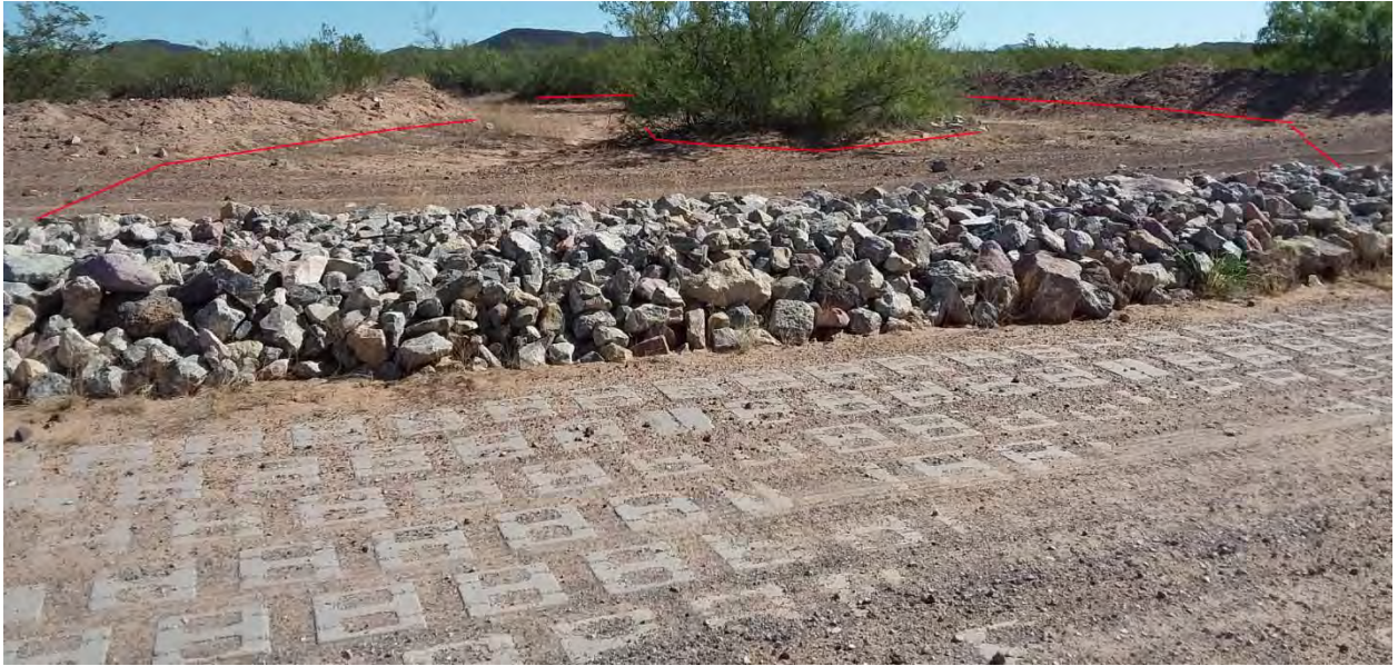
Figure 14 Photo point D1, looking upstream into the U.S.
