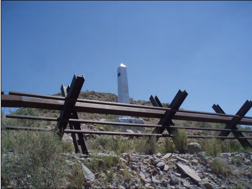
Figure C11. Overview of International Border Monument 14 facing south-southwest.
