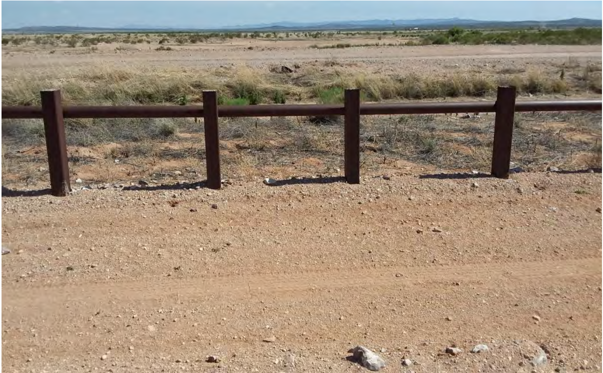
Figure 55 Photo Point R1, looking downstream into Mexico.
