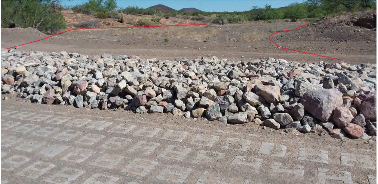
Figure 17 Photo point E1, looking upstream into the U.S.
