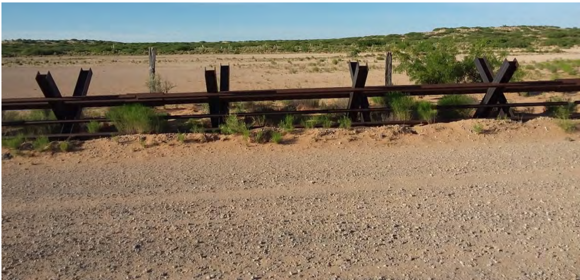
Figure 6. Photo point A2, looking downstream into Mexico.
