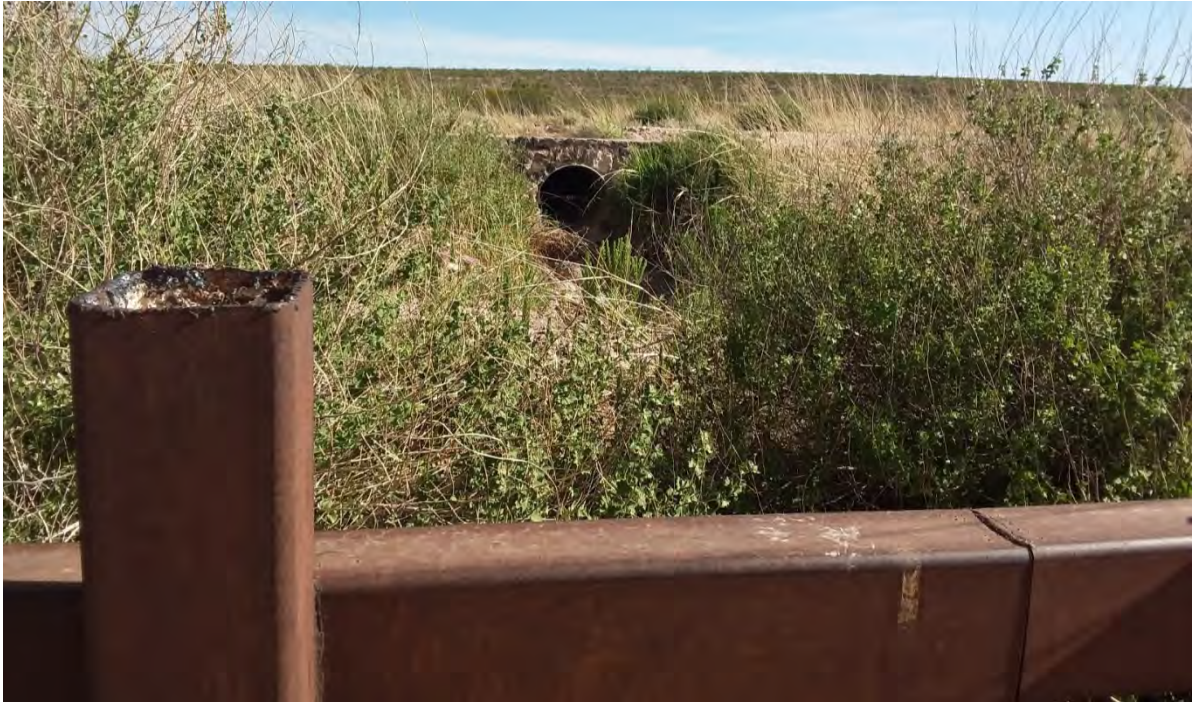
Figure 38 Photo Point L1, looking upstream into Mexico
