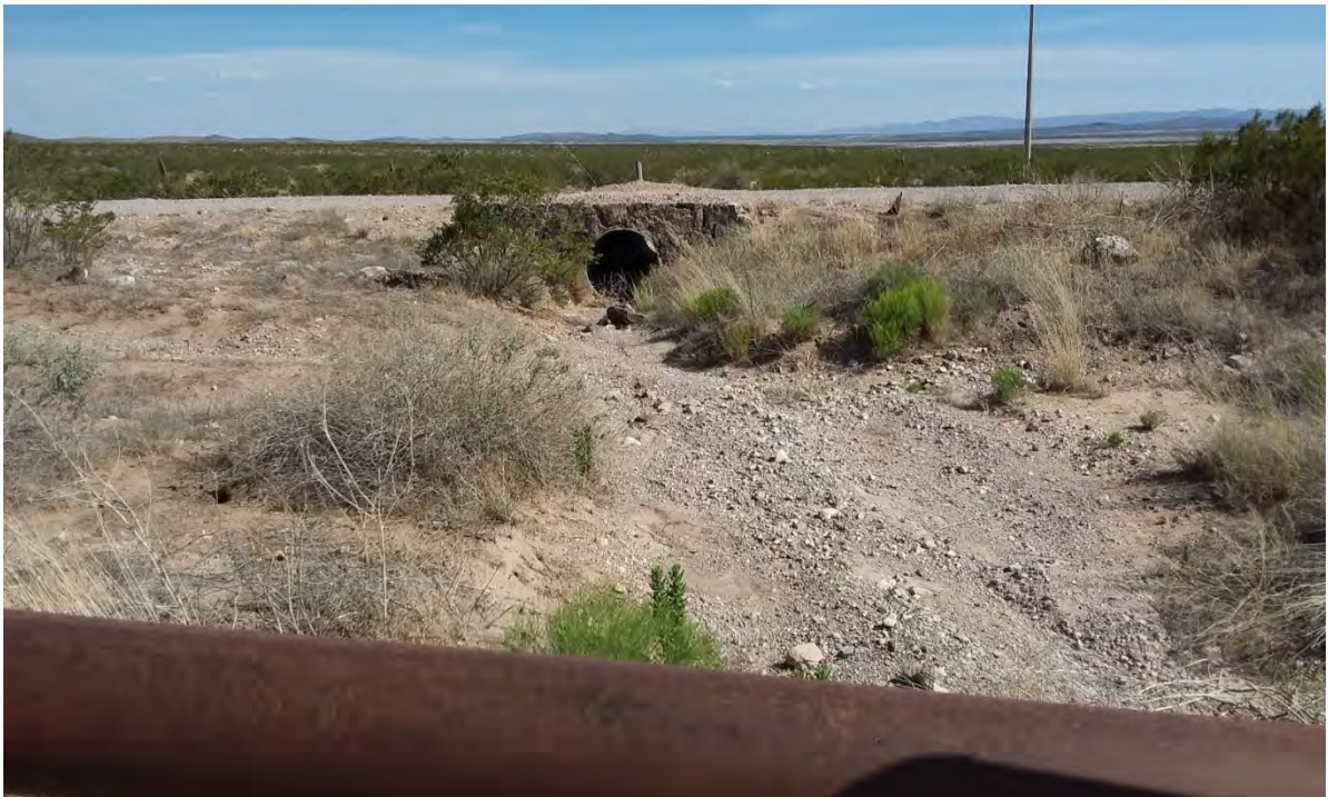
Figure 51 Photo Point P2, looking downstream into Mexico.
