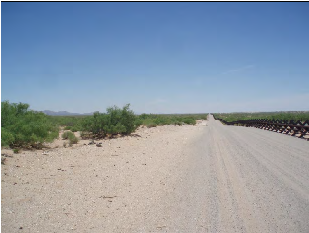
Figure 19. Overview of the typical condition on the APE along the Roosevelt Reservation western segment.
