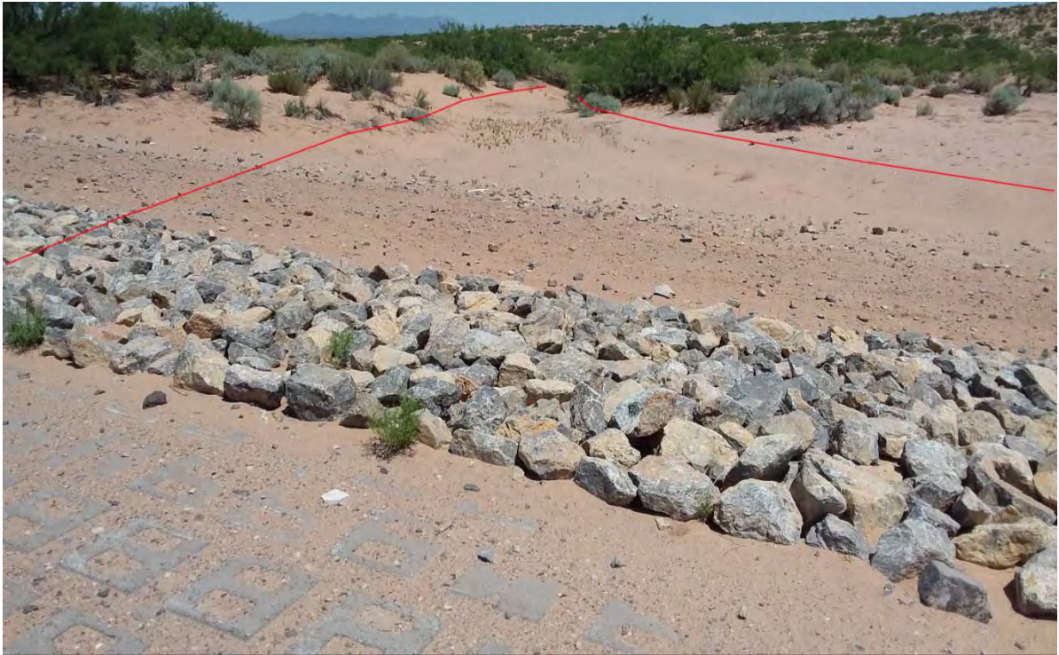
Figure 31 Photo Point J1, looking downstream into the U.S.
