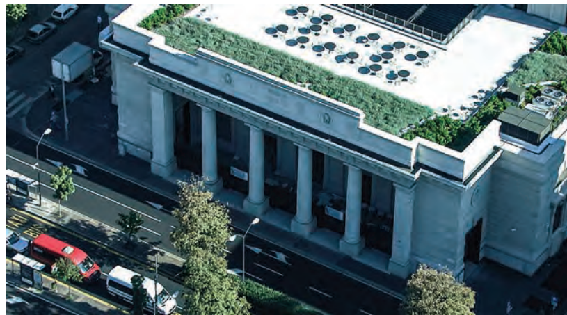
Historic seat of Royal Post, Aporti Palace has now become a new office building.
