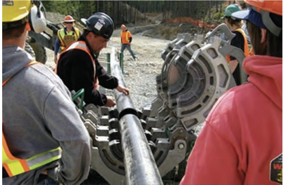
Polyethylene piping was laid across the site
