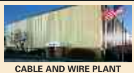
CABLE AND WIRE PLANT
