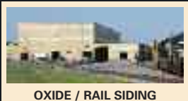
OXIDE / RAIL SIDING
