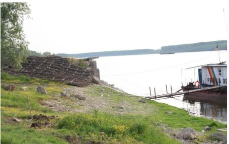
Figure 3.1.1.7 - Fascine mattresses temporarily stored for the purpose of water transport to another location
