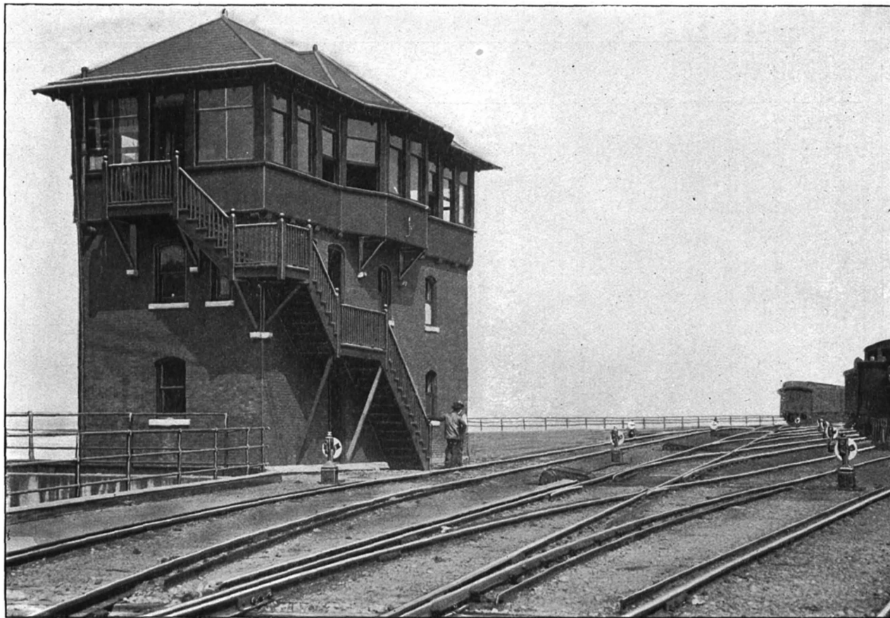
EXTERIOR VIEW OF TOWER AT LA SALLE STREET, CHICAGO.
