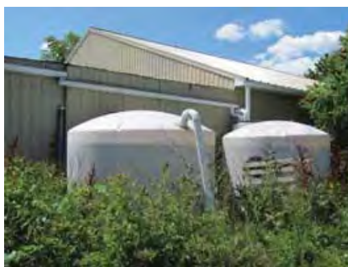
Fig. 2. A side view of the Horticulture Services Building (Macdonald Campus, Sainte-Anne-de-Bellevue, QC, Canada), two 2500-gal (9463.5 L) polyethylene water tanks, and the sheet metal roof directed using 4-inch (10.2 cm) aluminum eaves troughs with downspouts.
