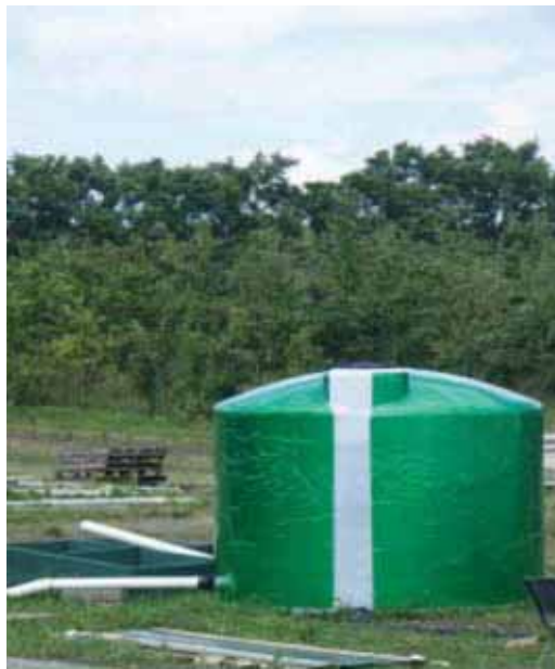
Fig. 4. A 2500-gal (9463.5 L) polyethylene water tank at the Horticulture Services Building (Macdonald Campus, Sainte-Anne-de-Bellevue, QC, Canada) wrapped with metallic green wallpaper to reflect almost all the sunlight, preventing any algal blooms.
