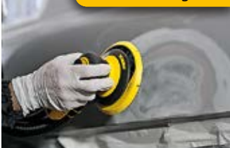
Paint removal / Feather edge
