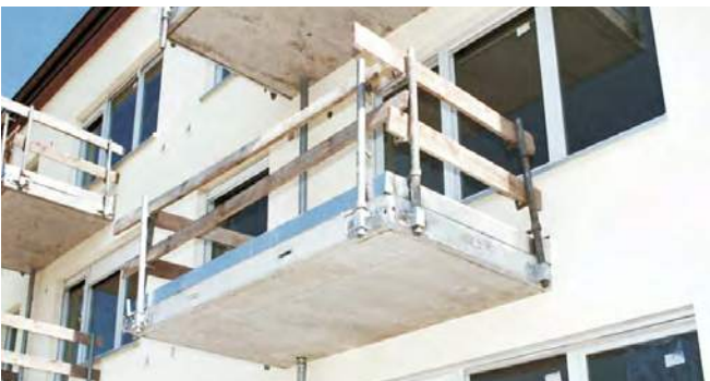
Used to secure safety rails during the construction phase
