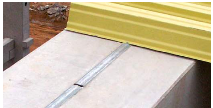
Fixing of trapezoidal sheet metal roof element
