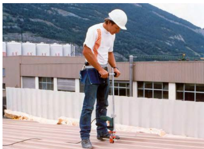
Fixing trapezoidal sheet metal using self-drilling screws
