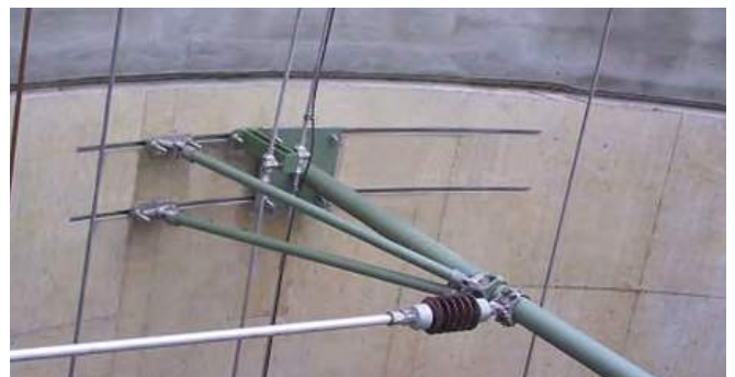
Fixing of overhead cables in railway tunnels
