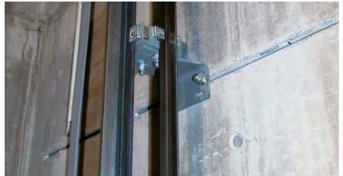
Fixing guide-rails with HALFEN Channels
