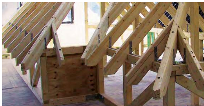
Timber pitched-roof construction
