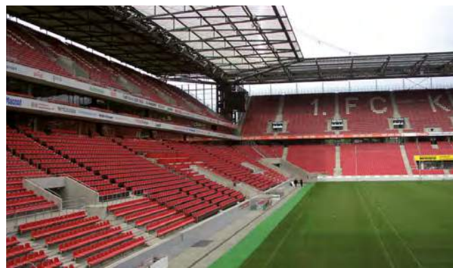
Fixing of safety rails, Rheinenergiestadion Cologne
