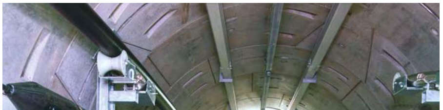
Curved HALFEN Cast-in channels in tunnel segments
