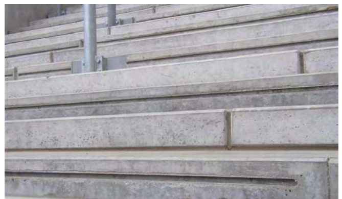
Fixing of safety rails, Rheinenergiestadion Cologne
