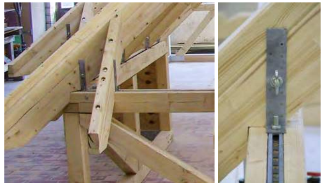
Timber roof construction with HALFEN HNA Fixing straps
