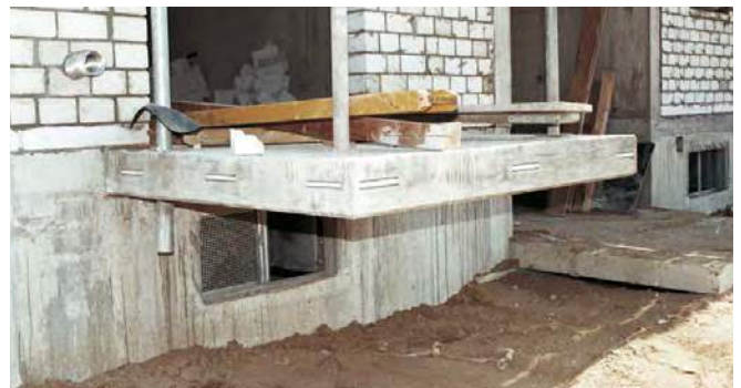
Cast-in HGB Channel, residential building
