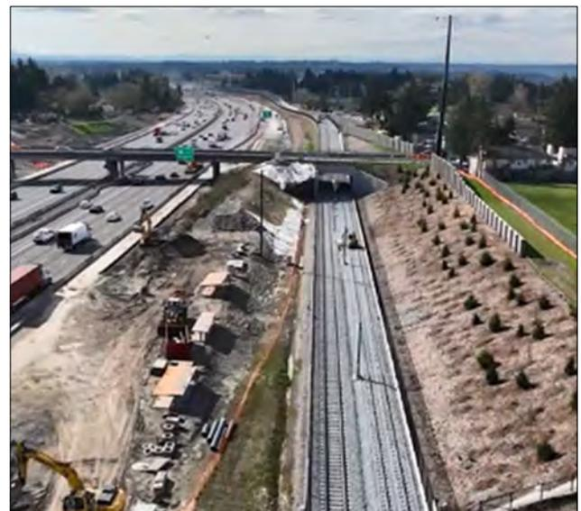
Ballasted track and traction power pole installation started
