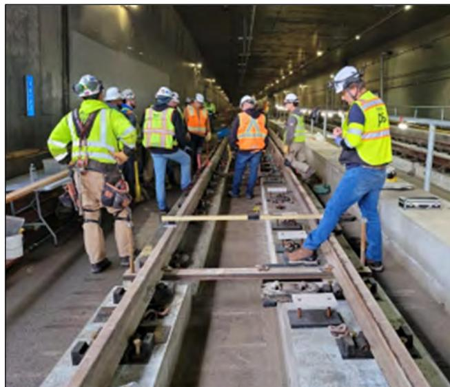
Crews inspecting final track alignment in Mt. Baker Tunnel
