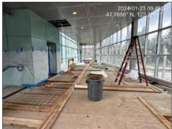
185th station pedestrian overcrossing concrete formwork
