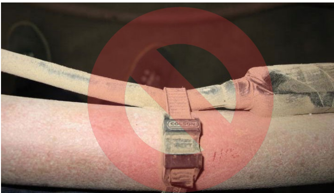
Figure 17. Do not use Zip-Ties Directly on Cables
