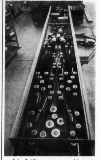
Rube Goldberg appearance of facer-canceller belies its 24,000-letter-per-hour capacity. System of photocells controls belt drives moving letters through the machine to cancelling heads in foreground. Metered and unstamped mail is deflected into tray which is shown at the right of machine.
