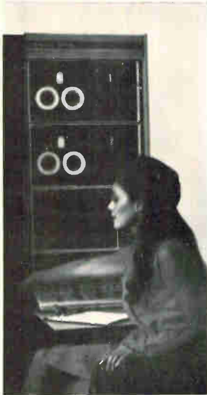
Family resemblance. Operator console combines features of PDP and LINC series. The upper banks of switches are for loading instructions and data manually; those below are for executing special functions.
