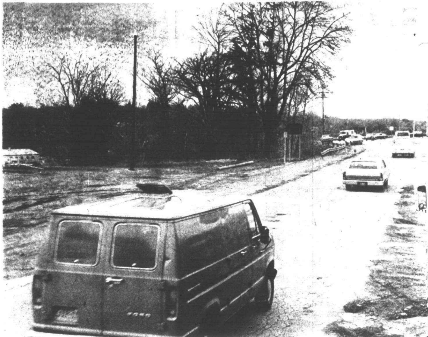
The curve at Northville Road and Five Mile will be eliminated this year by freeway construction. A bridge on Northville Road will begin at the north end of the Plymouth Hilton and carry over the
