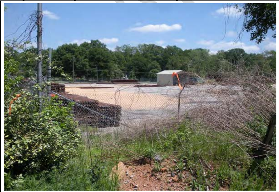
Photograph 14. View of Finding No. SW-4 (Former Woodworking Facility), facing north.
