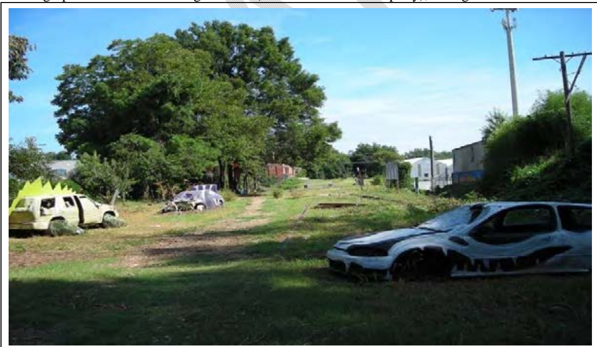
Photograph 28. View of Finding No. E-7 (Former Industrial Property), facing north. Inactive tracks extend from Memorial Drive up to Wylie Street.
