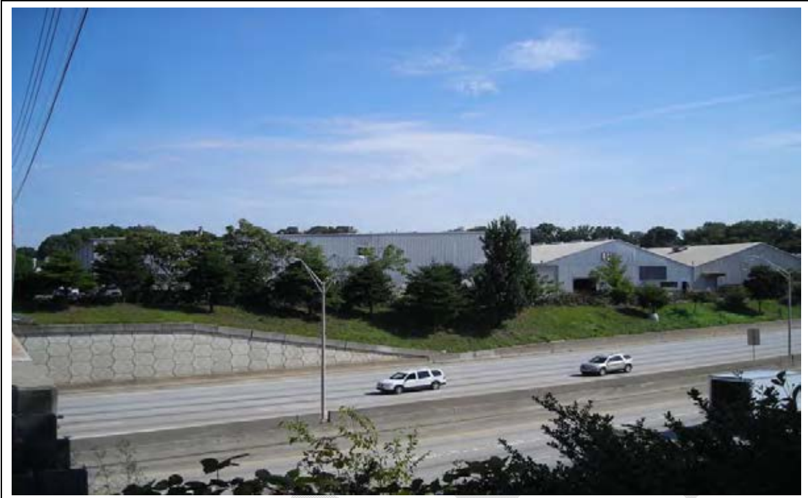
Photograph 27. View of Finding No. E-5 (Former Industrial Property), facing northeast.
