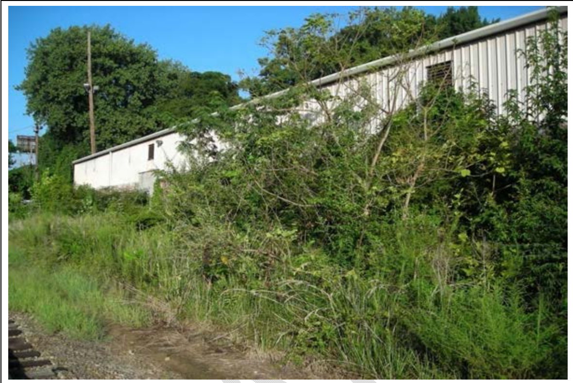
Photograph 21. View of Finding No. SE-14 (Unknown Lust), facing north.
