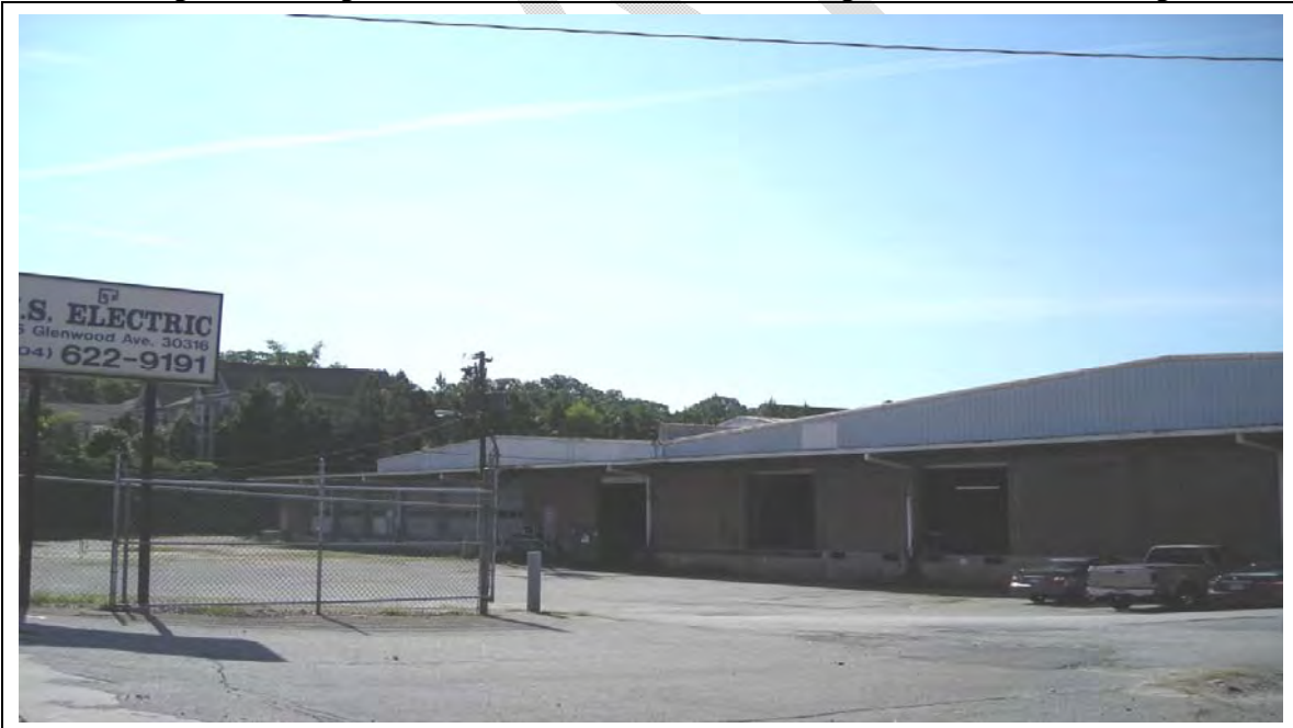
Photograph 26. View of Finding No. E-3 (Former Industrial Property), facing southeast. The BeltLine extends northward as the Bill Kennedy Way Overpass from here to Memorial Drive.
