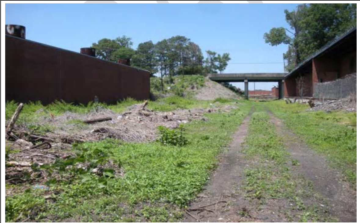
Photograph 8. View of subject site approximately 300 feet east of Lawton Street, facing west.
