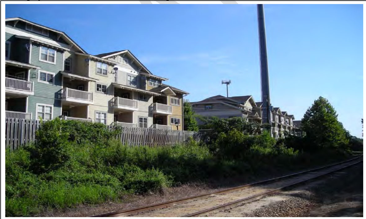
Photograph 24. View of Finding No. E-1 (Former Truck Depot), facing northwest. Finding No. E-2 (Former Industrial Property) is farther north.
