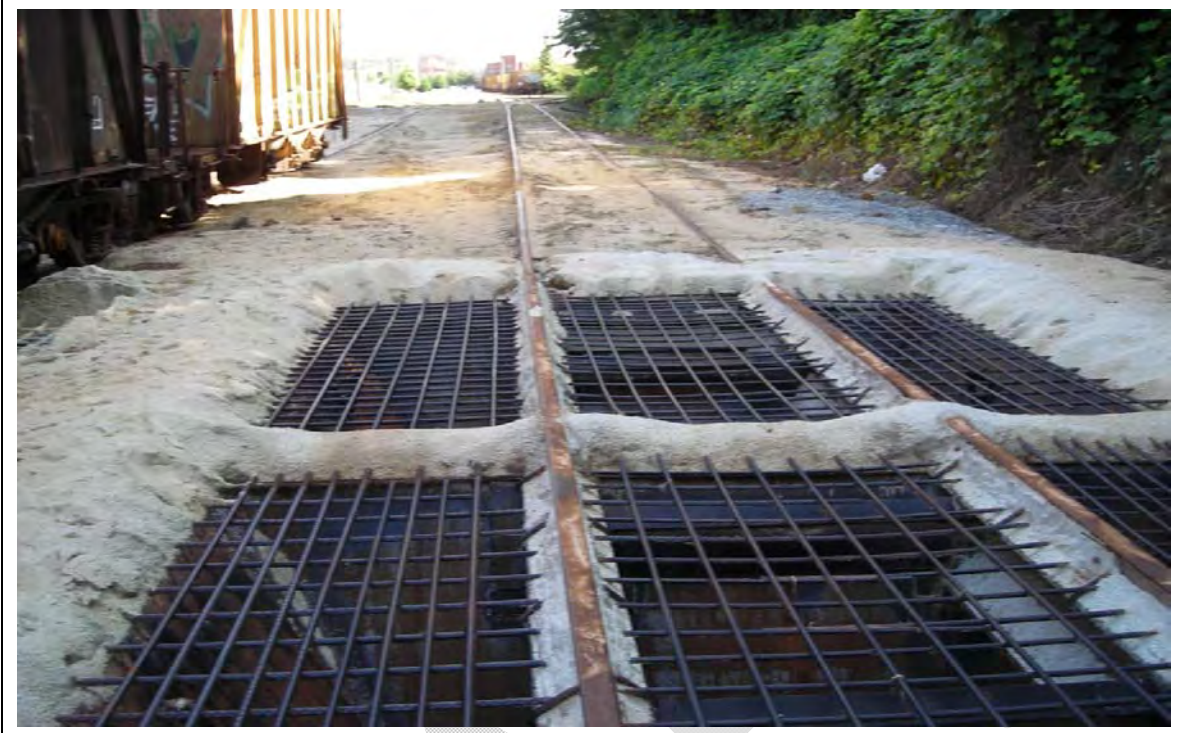
Photograph 25. View of active track portion of subject site approximately 100 feet north of Berne Street, facing north. The grated area on the tracks is for receiving raw materials at LaFarge.
