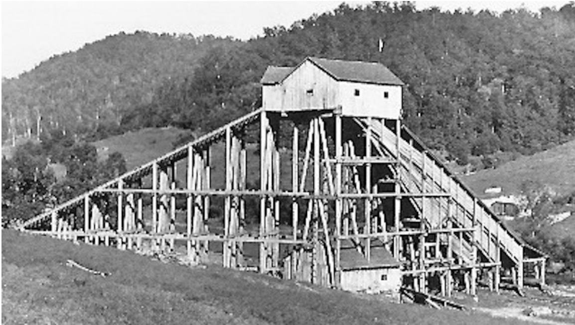
THE ORIGINAL TIPPLE AT VIRGINIA CITY WAS OF THE STYLE USED IN THE PENNSYLVANIA ANTHROCYTE FIELDS, AND WAS CALLED A 'BREAKER' - THE COAL CARS FROM THE MINE TO THE LEFT WERE PULLED UP THE RAMP BY CABLES BEFORE BEING DUMPED
