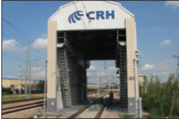
Figure 19.10 Automated Wheelset and Pantograph Inspection Site
