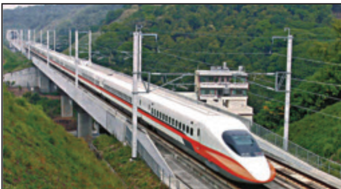
Figure 2.1 700T High Speed Trainset
