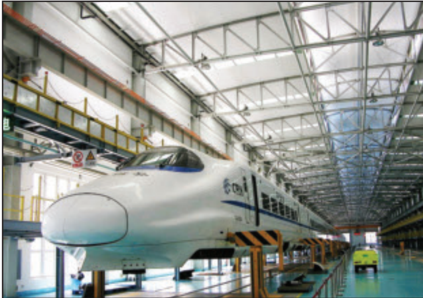
Figure 19.4 CRH Maintenance Depot Showing Trainset Lift/Bogies Removed
