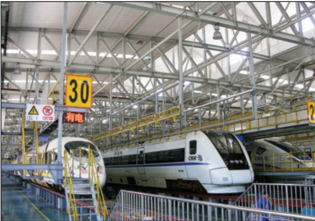
Figure 19.5 CRH Maintenance Depot Showing Three-Layer Working Platform
