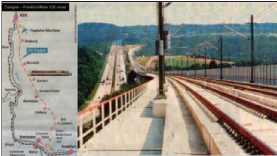
Figure 21.3 Wind Barriers on the Cologne-to-Frankfurt Line
