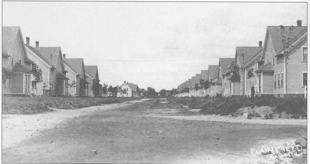
Figure 6-11. Lawton Mills housing in 1910. The Cote family may have lived in one of these units. Photo from Reference 5.
