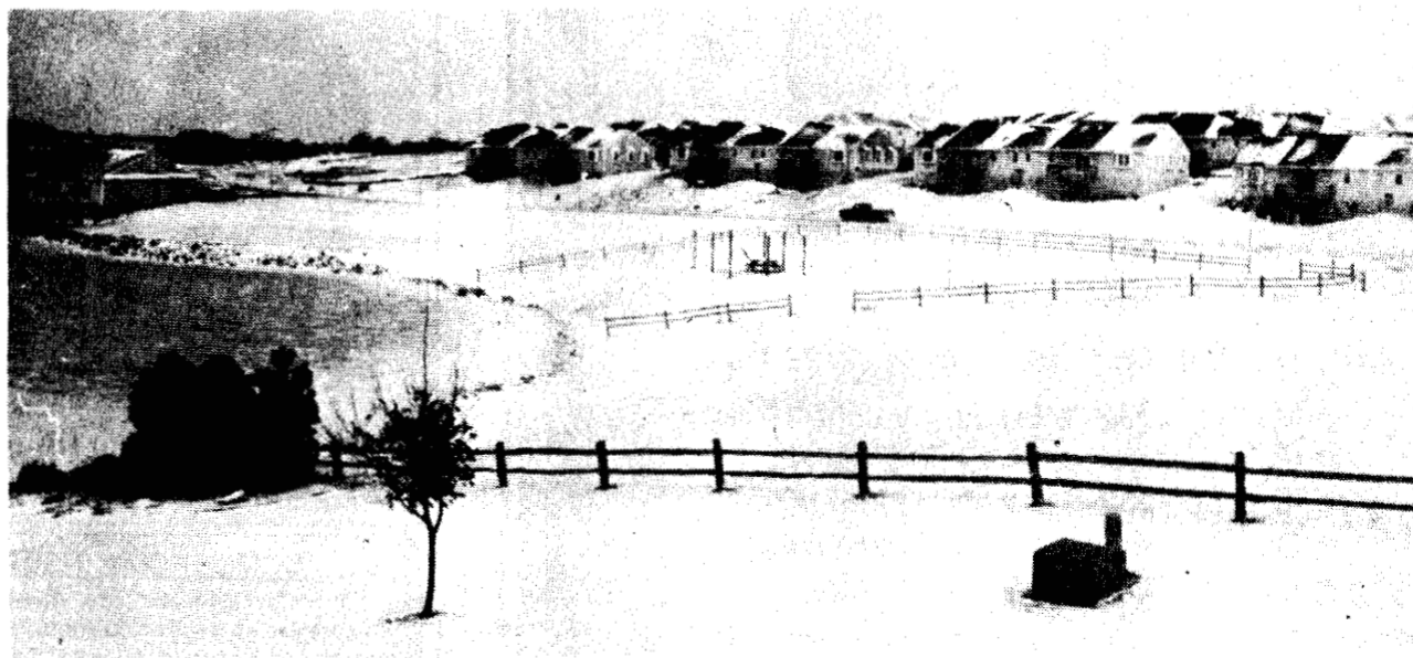
CONTINUED GROWTH AT Northwood Lake Condominiums (above) in Cass City accounted for some 70 percent of new construction permits issued in the village this year.
