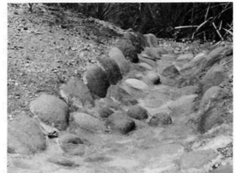
River boulders used to construct a dry, stable walking surface.
