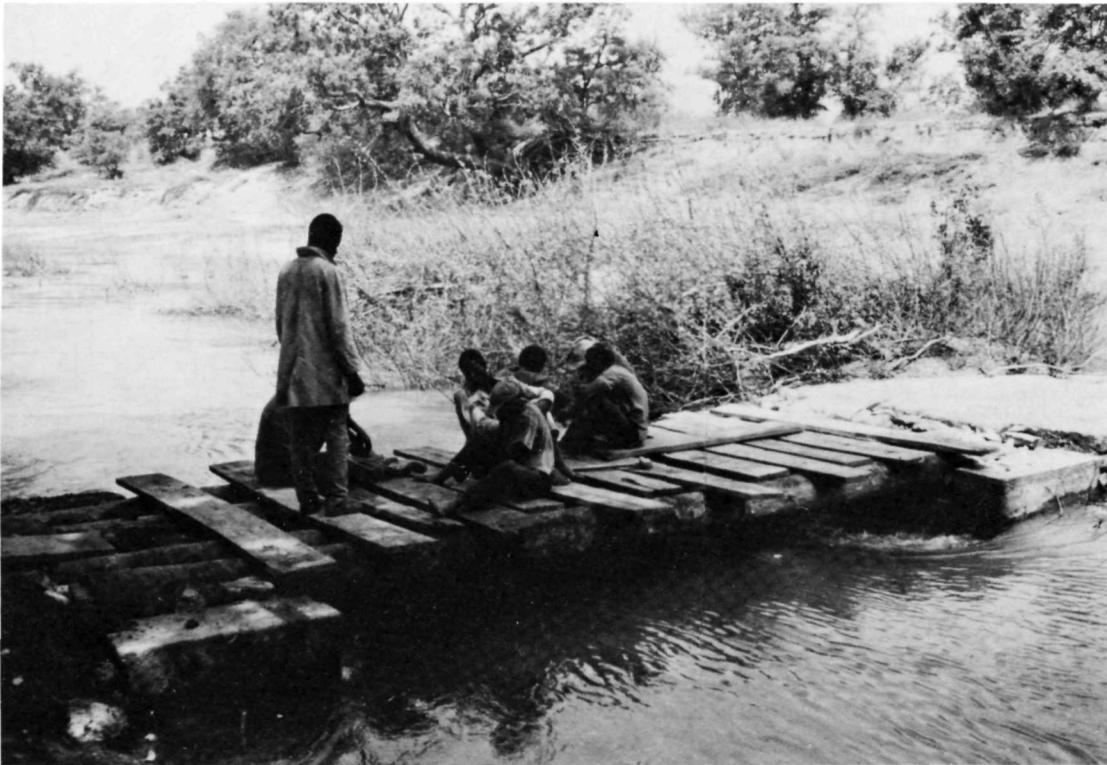
This Pendjari river bridge was built almost entirely of local materials by local labor.
