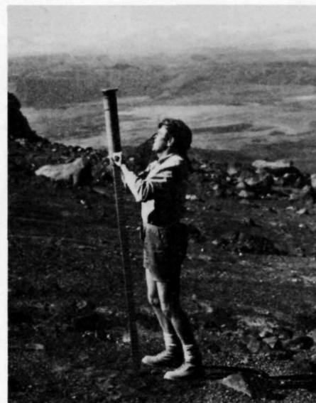
Installing track poles across open ground.
