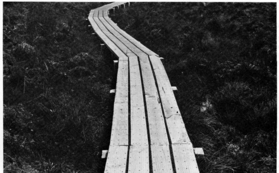
A board walk across an alpine bog. Curves reduced the visual impact.
