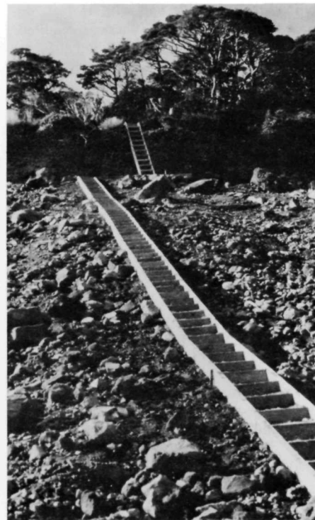
Boxed steps up an unstable slope.
