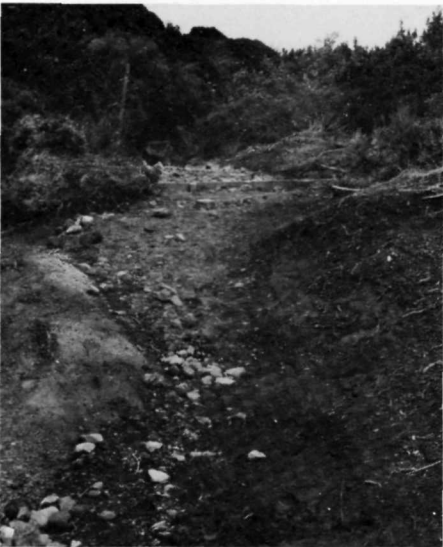
Unless tracks are adequately drained, erosion could develop into a major problem.
