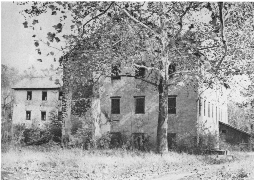
A remnant of Atsion's past. Rumored to have been a monastery, this huge stone building once employed 170 workers and variously served as cotton mill, paper factory and cranberry-packing plant.
