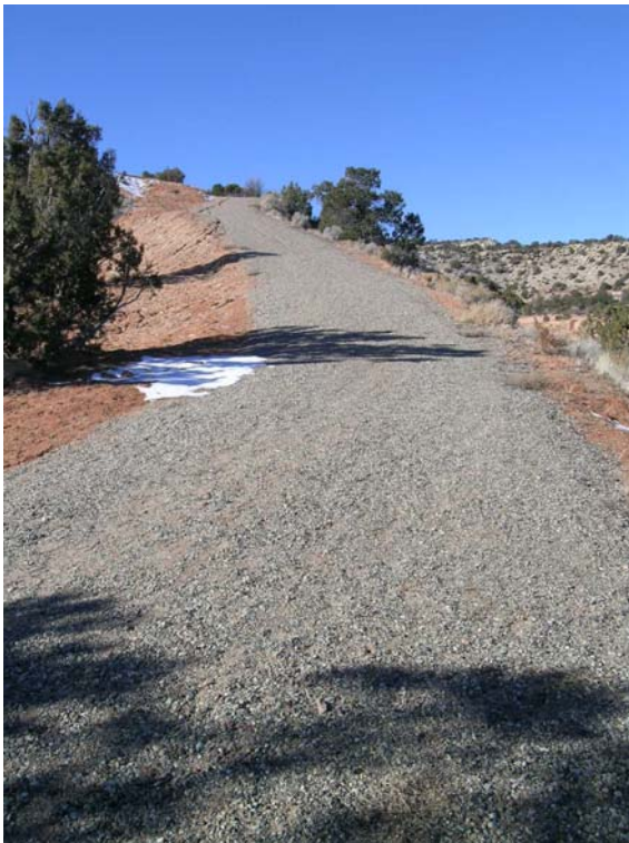
Gravel Road in Monnument
