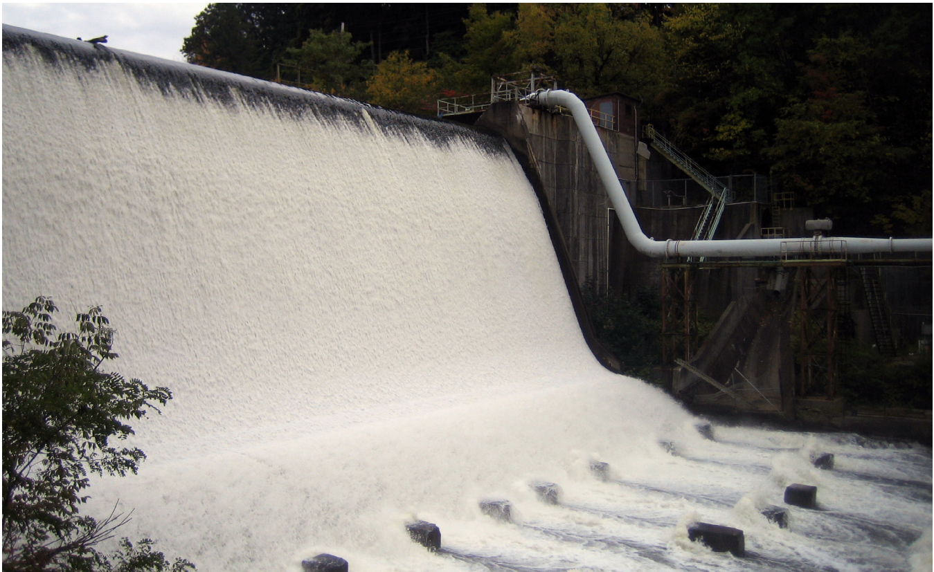
Figure 27. Photograph of the dam at the Gorge Metropark. The dam was originally constructed to support hydroelectric power generation and was later used to provide cooling water for a coal-fired power plant (now razed). Today, such features impede natural river flow and pose water quality hazards. Several park dams have been removed or are being considered for removal, including this dam. Photo by Trista L. Thornberry-Ehrlich (Colorado State University) taken in autumn 2009.
