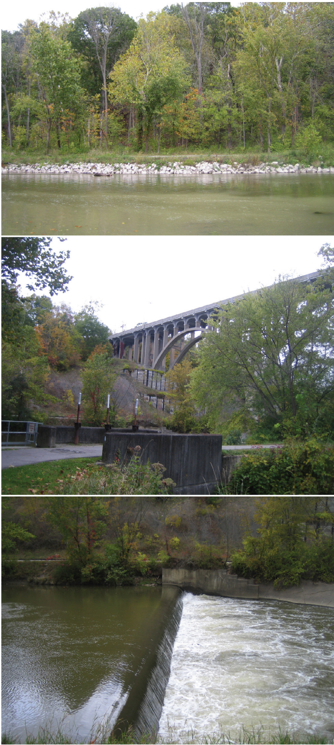
Figure 26. Photographs of water-control features. Riprap (top image) along was installed on shorelines to mitigate erosion and lateral meandering. Locks (middle image) and dams (bottom image) were constructed in many locations along the river. Photographs by Trista L. Thornberry-Ehrlich (Colorado State University) taken in autumn 2009.
