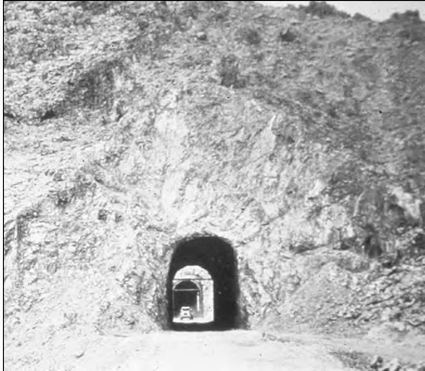
Figure 10. Vehicles had access to Hoover Dam through the U.S. Government Construction Railroad tunnels. Built in 1931, the railroad aided in the construction, maintenance, and repair of Hoover Dam. Courtesy of the National Park Service.
