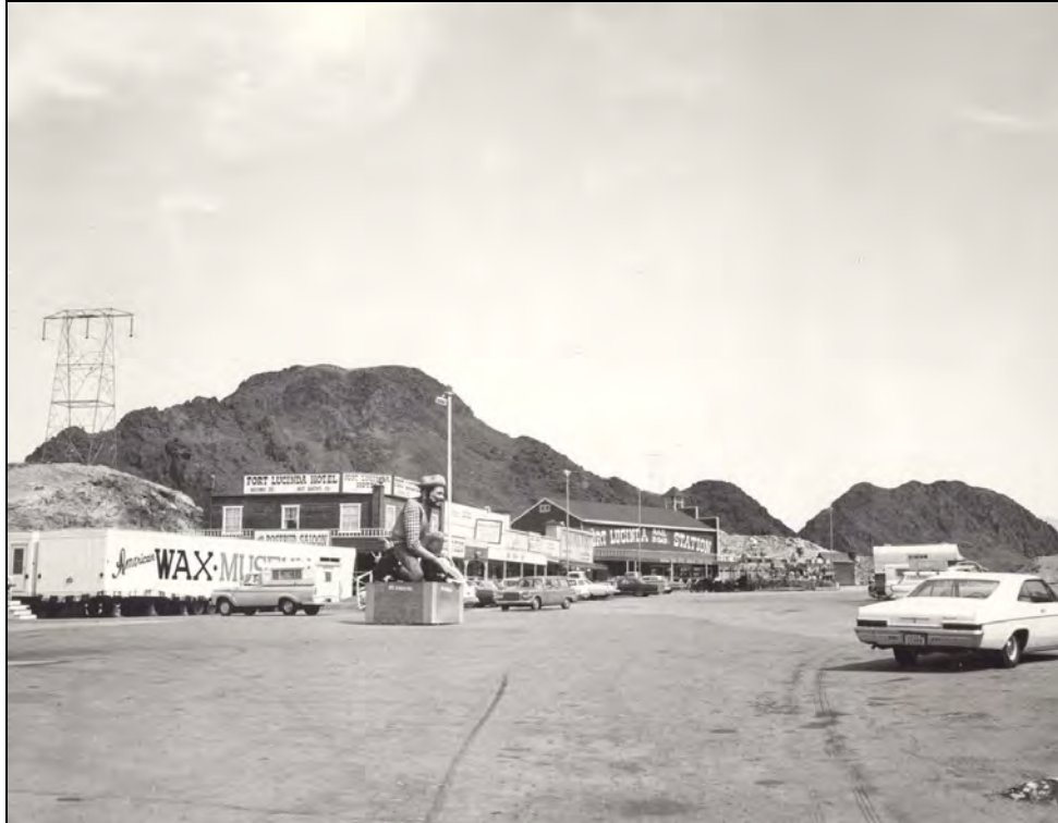
Figure 12. The Gold Strike Inn was a fixture on the park's boundaries, typical of the kinds of uses that required constant vigilance by the National Park Service. Courtesy of the National Park Service.
