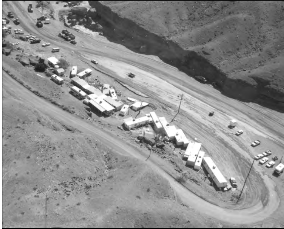
Figure 25. In 1974, the Nelson Landing area was devastated by the worst flood in park history. This photo from the air, taken within days of the tragedy, reveals the destruction of the little community.
