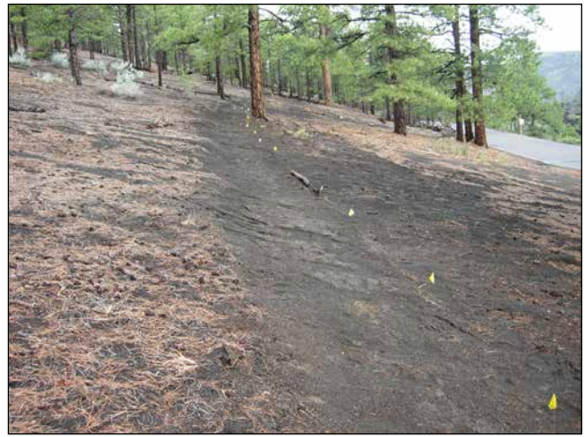
Figure 4.5.4-4. New trail ascending Lenox Crater follows contours and is therefore less susceptible to erosion. Photo Credit: NPS/P. Whitefield.
