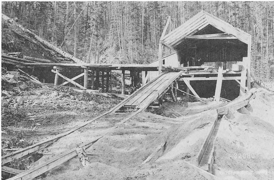
Trail Creek Sawmill and pipe conveying water to wheel. Gallatin N.F. - 1902.
