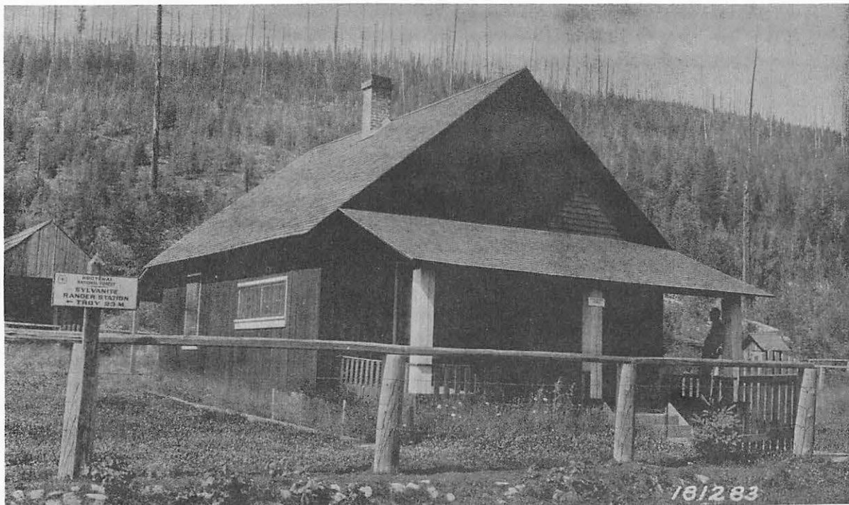
Sylvanite Ranger Station, Kootenai National Forest, August 1923. Area behind building was burned over during 1910 fire.
