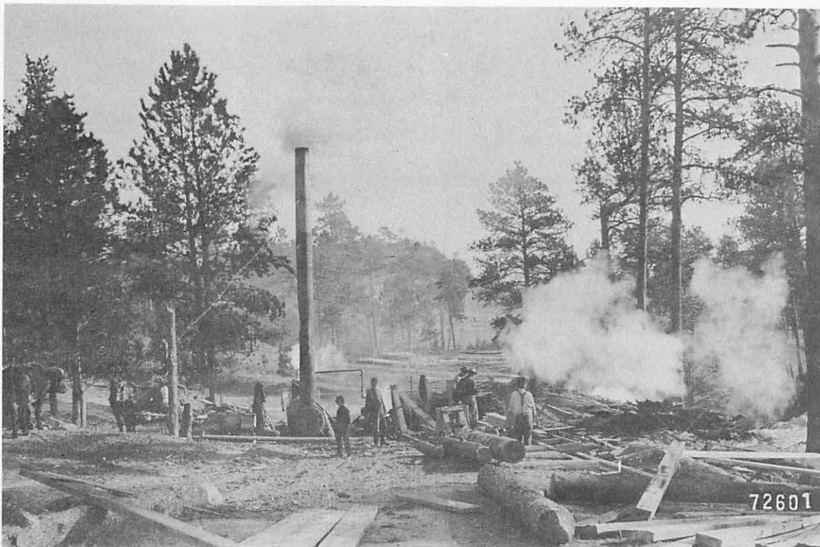
Sioux N.F., Custer County, Montana - November 22, 1907 - Hall's Sawmill operating under payment in connection with sale. Note no spark arrester on stack.
