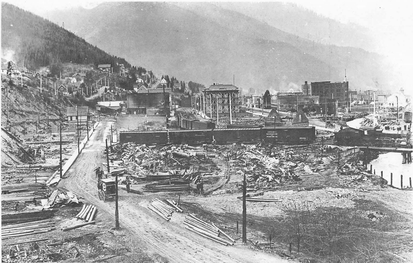
Wallace, Idaho, after the 1910 fire. On this terrace at Wallace every house was burned - about 200 in all.
