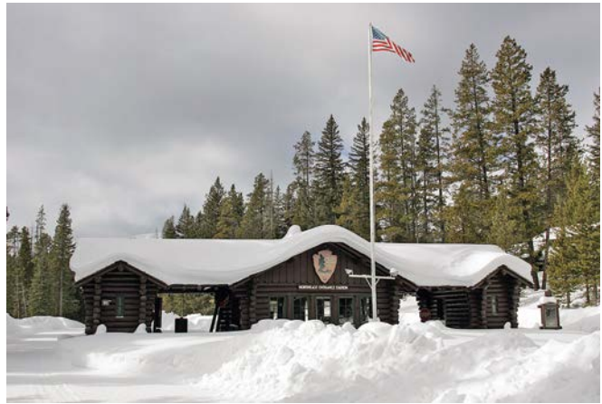
Northeast Entrance station is considered "the best of its type remaining in the National Park Service."
