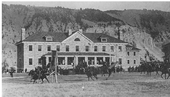
Albright Visitor Center, part of the Mammoth Hot Springs Historic District and Fort Yellowstone Historic Landmark District, housed the first "information office" (visitor center).
