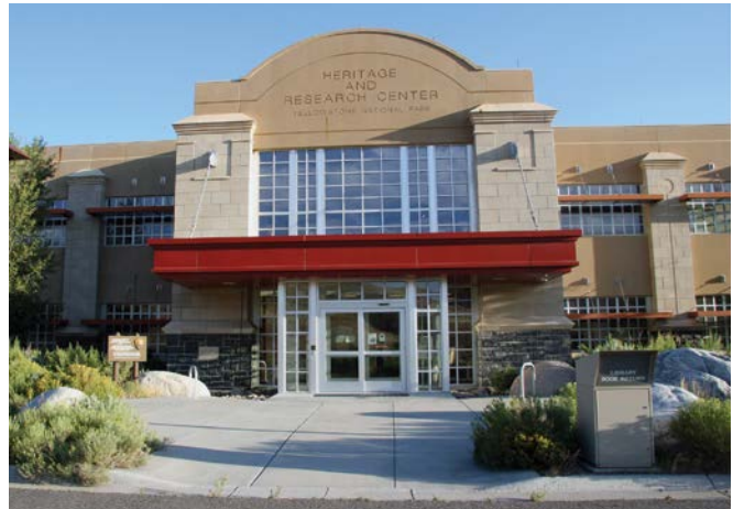
The Heritage and Research Center houses Yellowstone’s museum collection, archives, and research library.
