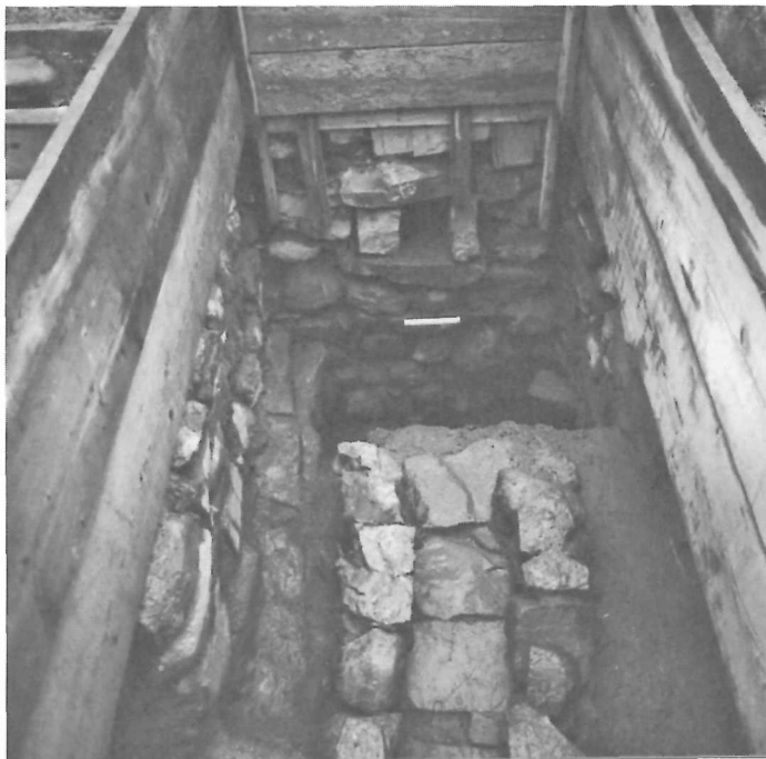
44 North curtain, mouth and portion of the drain used to draw off overflow from the well dug in the middle of the yard in about 1760.
