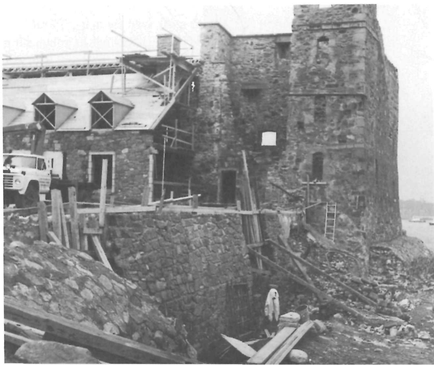
57 Restoration work on the north curtain.
