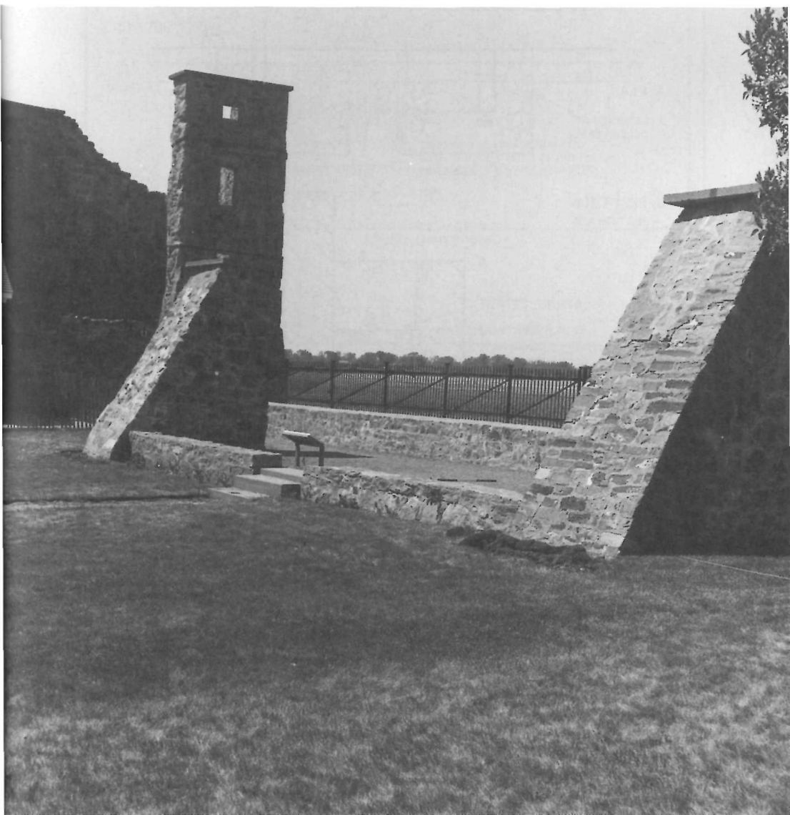
40 General view of the north curtain before excavations.
