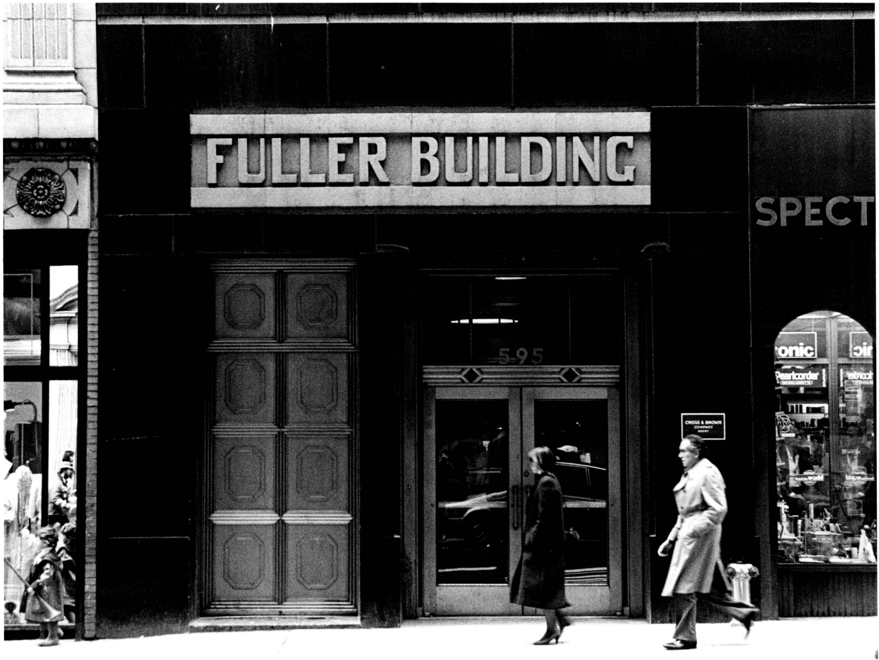
THE FULLER BUILDING Madison Avenue Entrance
