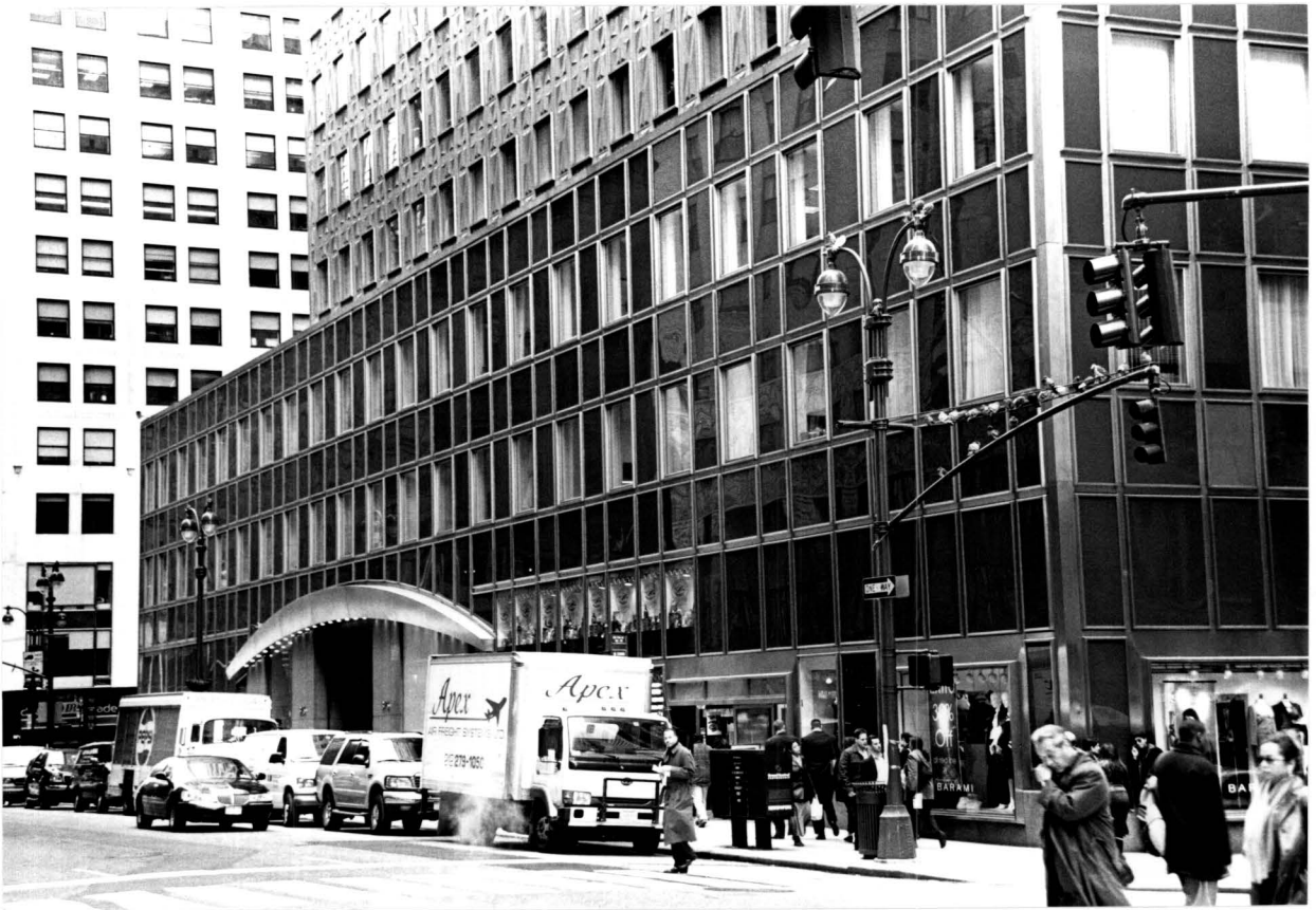
Socony-Mobil Building Lexington Avenue facade
