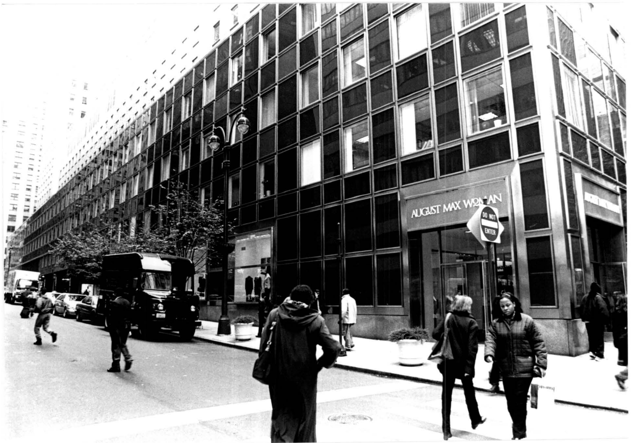
Socony-Mobil Building 41 st Street facade, looking west from Third Avenue Photos: Carl Forster
