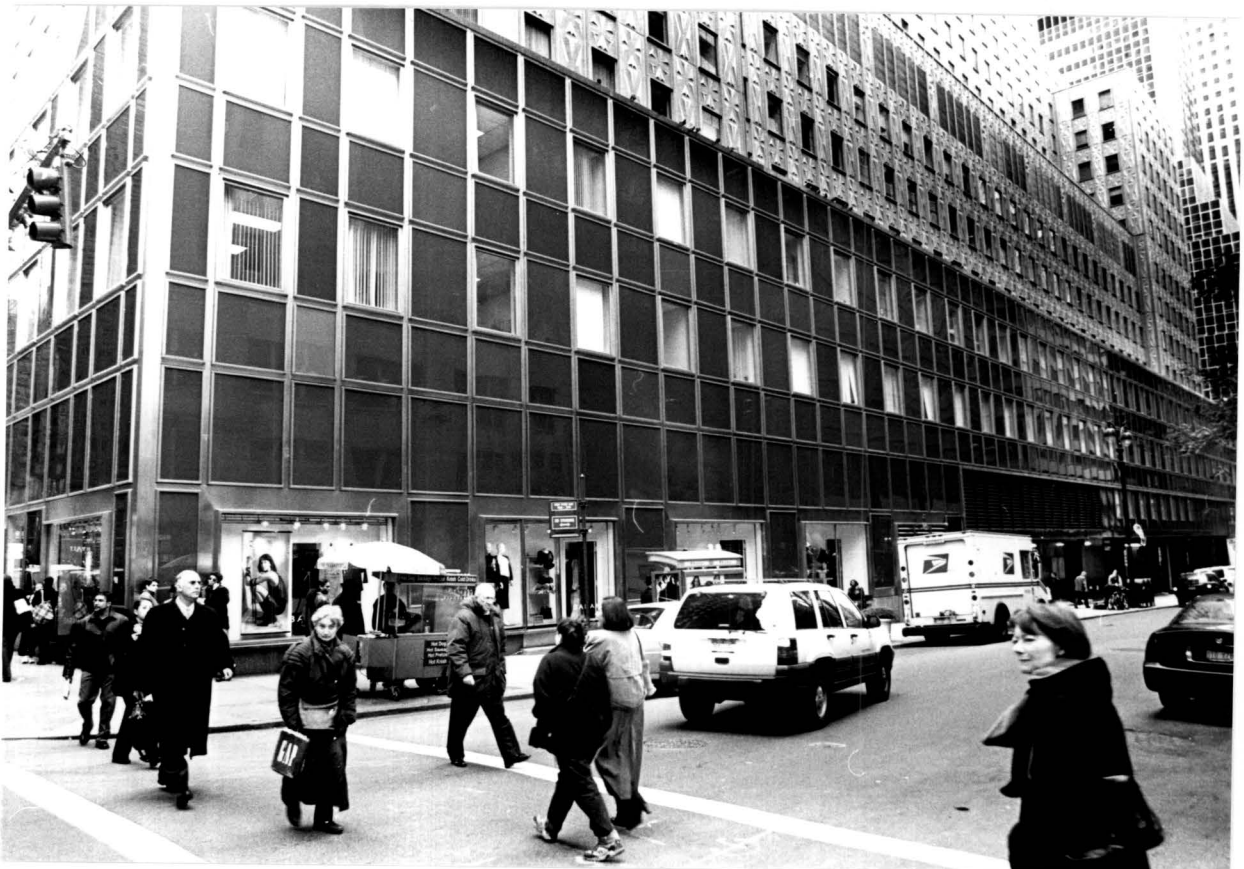
Socony-Mobil Building 41 st Street facade, looking east from Lexington Avenue Photos: Carl Forster
