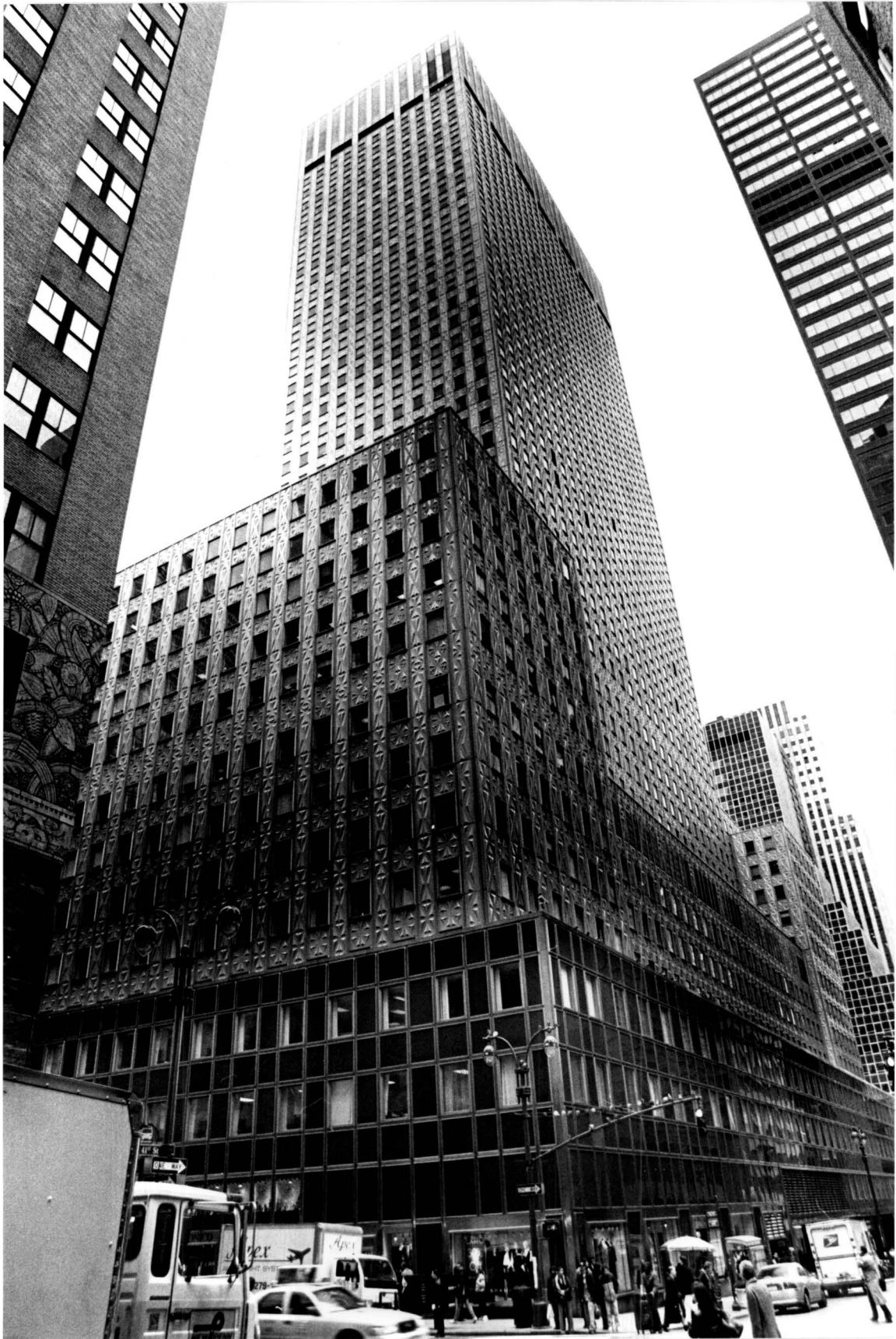
Socony-Mobil Building 150 East 42 nd Street corner of Lexington Avenue and 41 st Street Photo: Carl Forster
