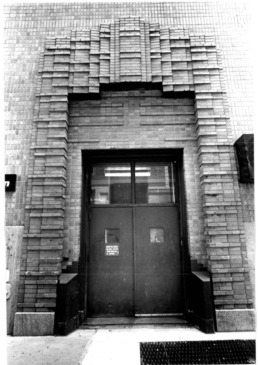
Service entrance, Bridge Street
