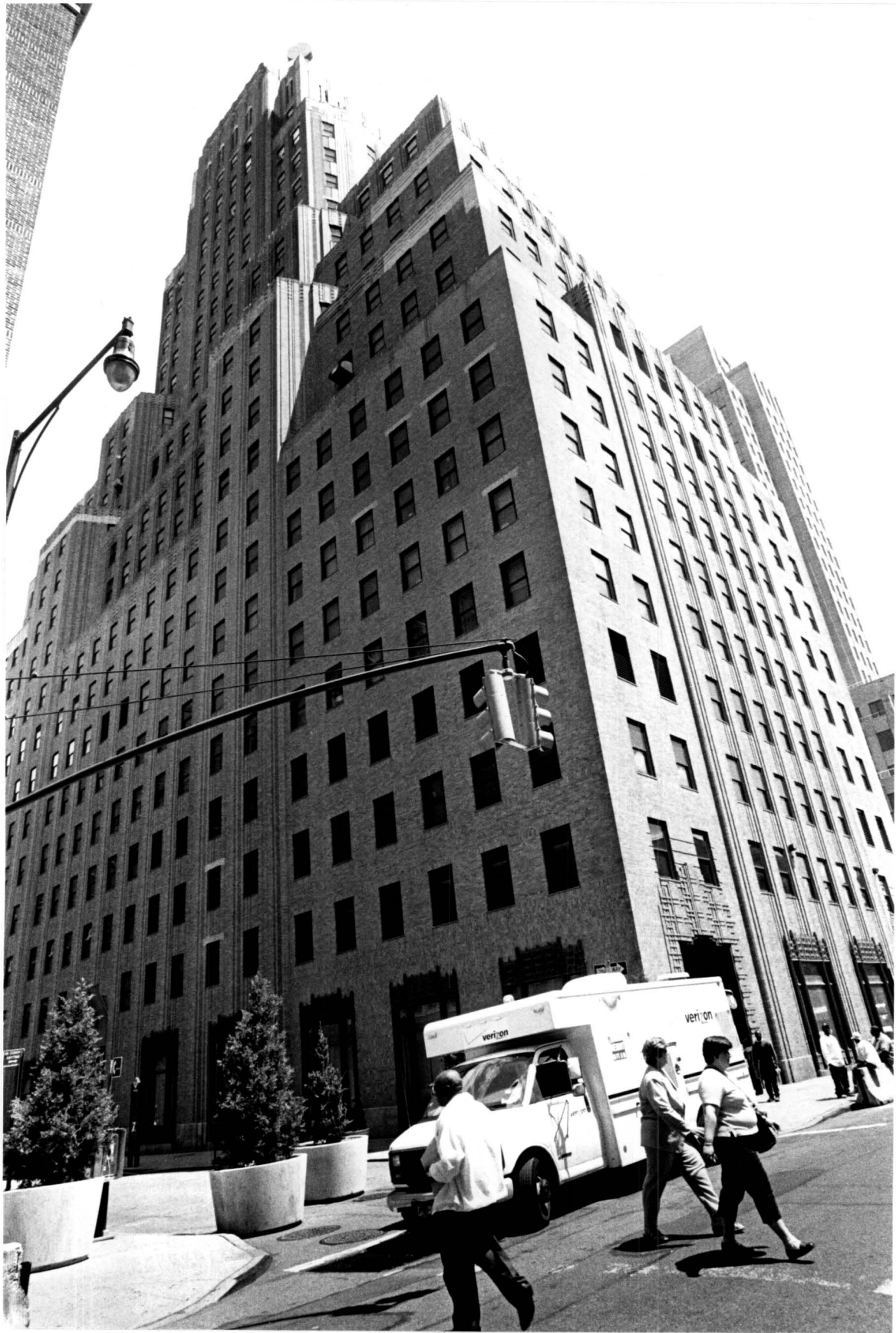
(Former) Long Island Headquarters of the New York Telephone Company 97-101 Willoughby Street, Brooklyn Bridge Street facade Photo: Carl Foster
