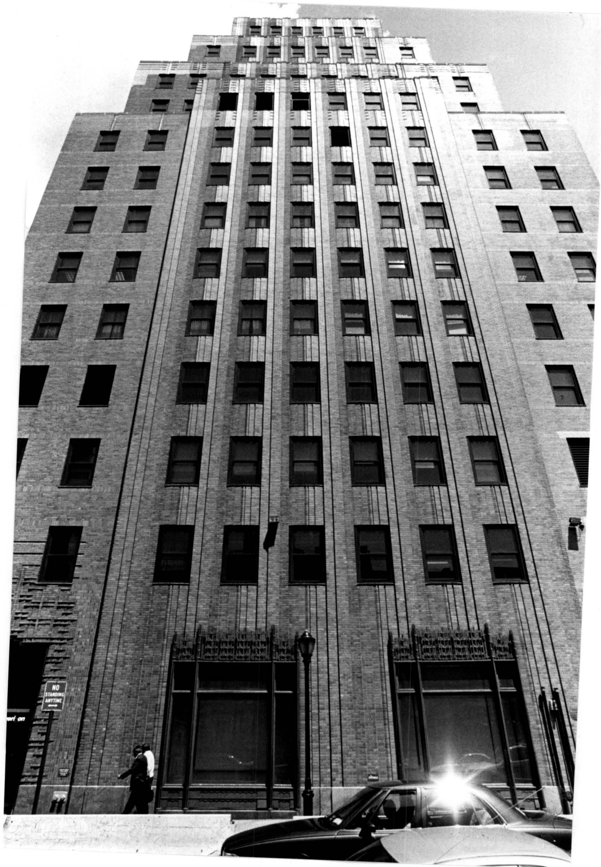
(Former) Long Island Headquarters of the New York Telephone Company 97-101 Willoughby Street, Brooklyn Willoughby Street facade Photo: Carl Foster
